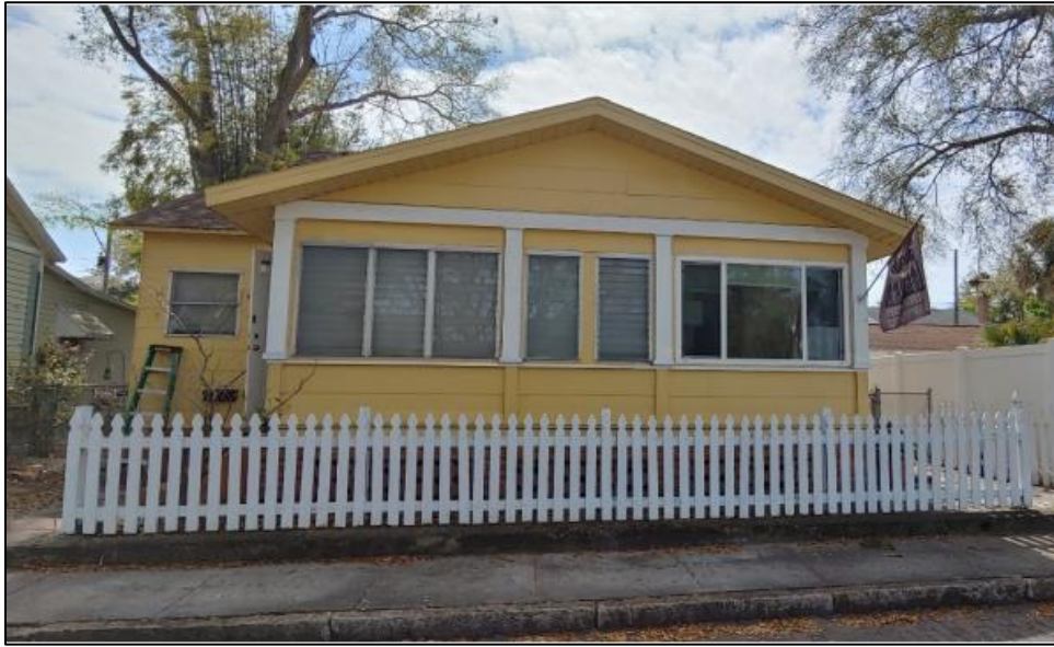
Figure 1: Front façade of subject property prior to construction.
