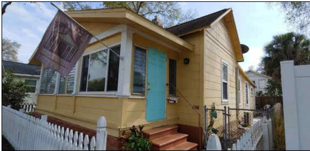
Figure 4: Front façade and side elevation, prior to construction
