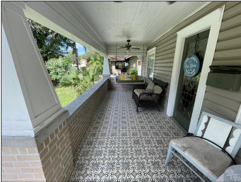
Figure 8: Detail of front porch.
