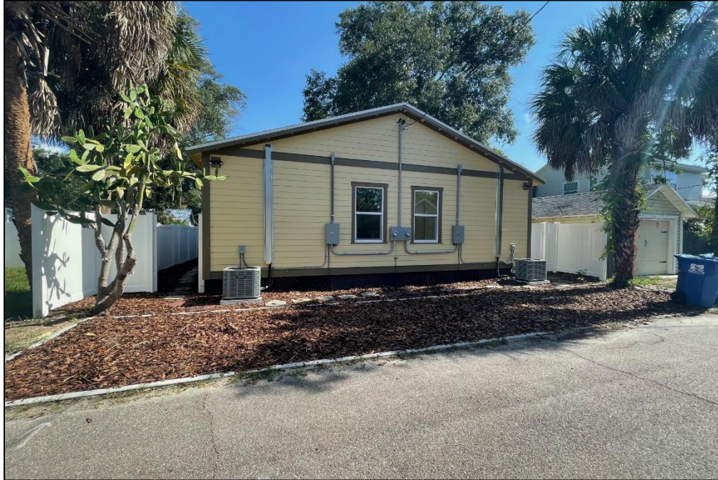
Figure 10: Rear elevation, after construction
