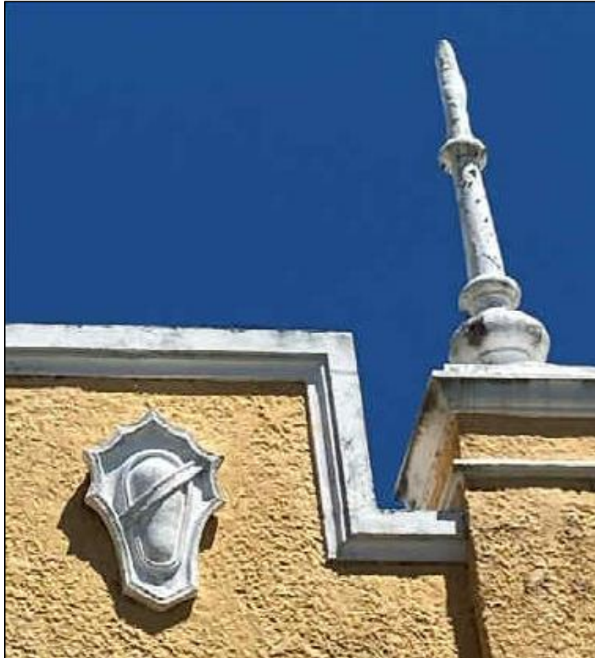
Figure 6: Closeup detail of pilaster
