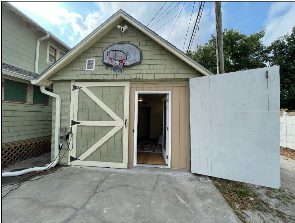
Figure 9: Garage with restored carriage door open
