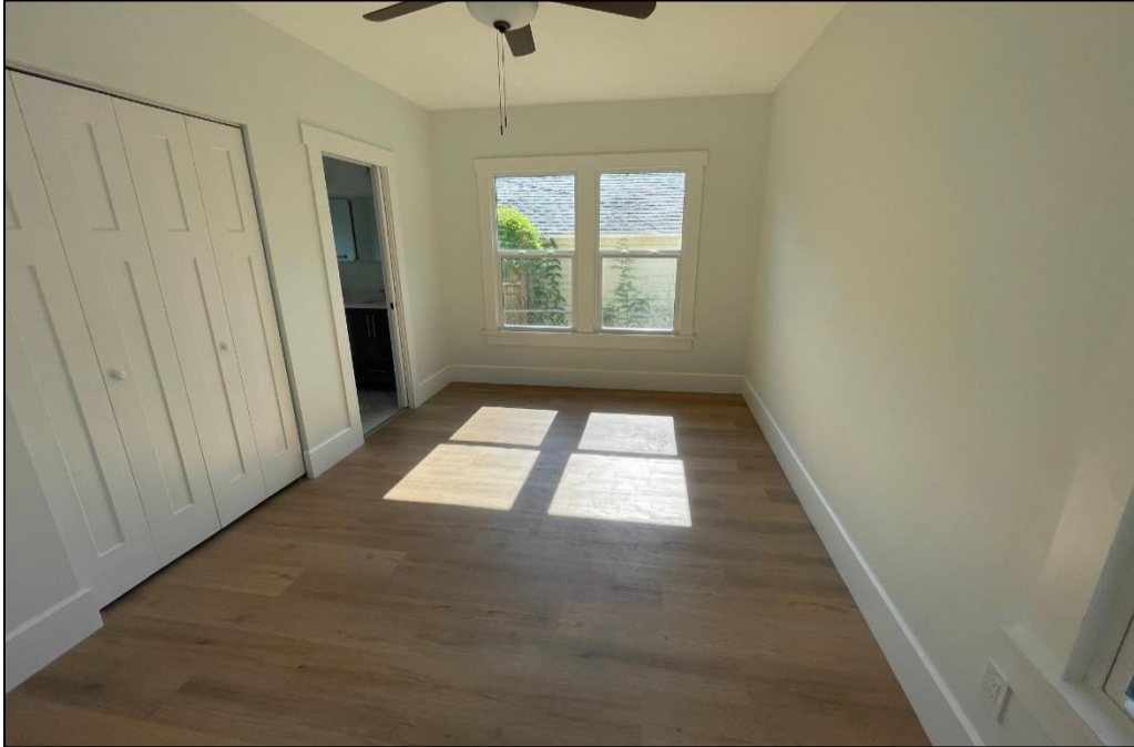
Figure 12: Bedroom in the addition
