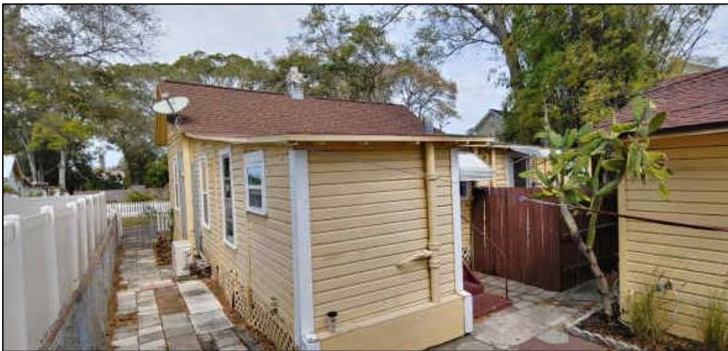
Figure 9: Rear elevation, before construction work
