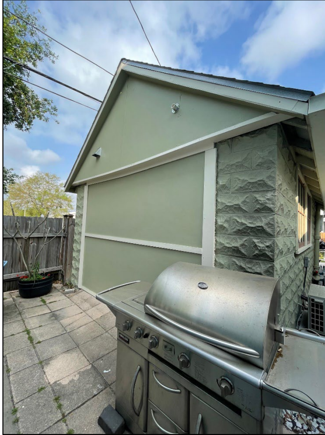
Figure 14: Rear of garage with wall repair
