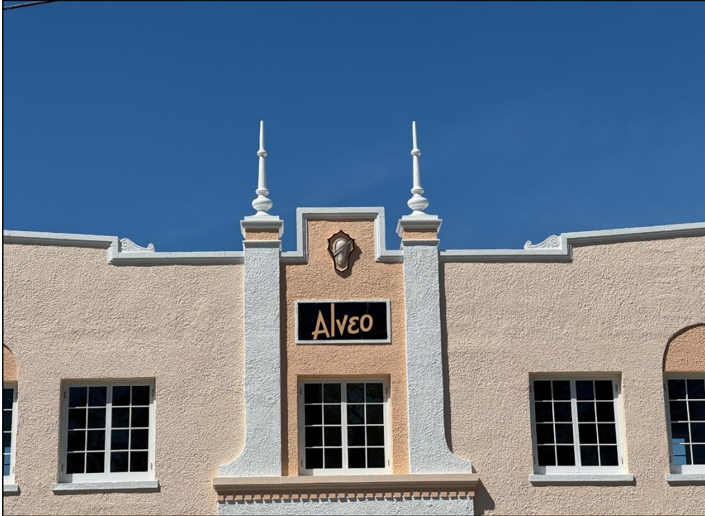
Figure 12: Detail of repaired pilasters, ornamentation, and parapet cap
