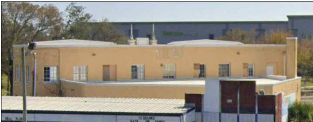
Figure 4: Rear elevation of building
