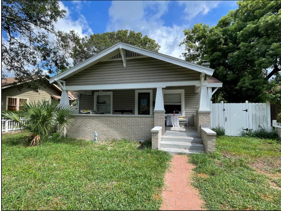
Figure 7: Front façade after reconstruction of porch columns, walls, and floors.
