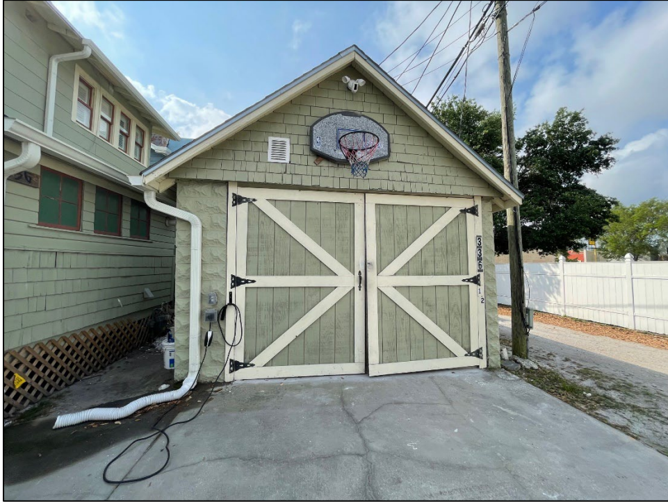
Figure 8: Front façade after conversion
