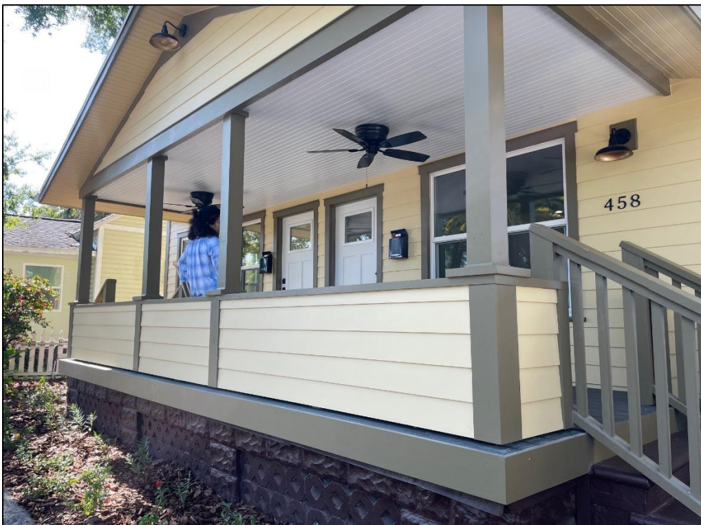
Figure 7: Another view of the front porch, after rehabilitation
