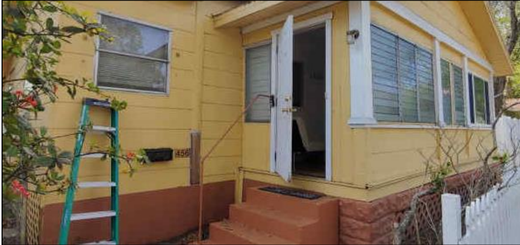
Figure 3: Enclosed front porch, prior to construction
