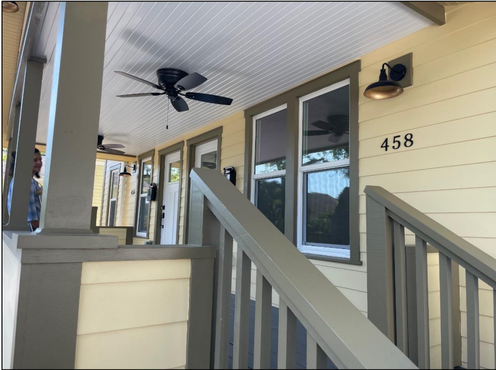
Figure 6: Front porch, after rehabilitation
