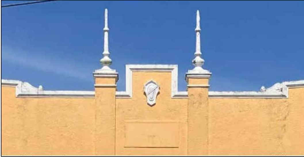
Figure 5: Detail of pilasters, parapet cap, and other ornamentation
