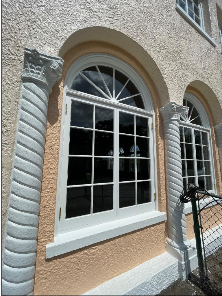
Figure 15: Detail of window reconstruction and ornamentation restoration
