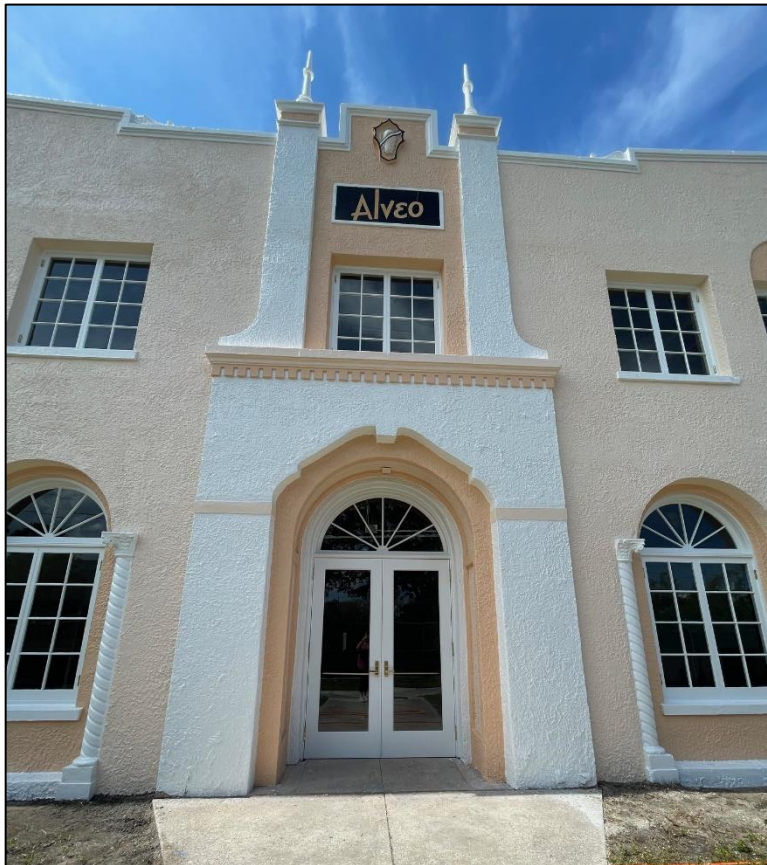
Figure 11: Front entryway restoration
