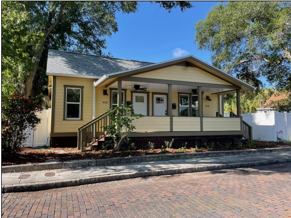
Figure 2: Front façade after rehabilitation.
