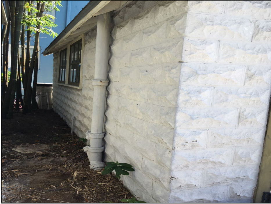
Figure 7: Side wall of garage building
