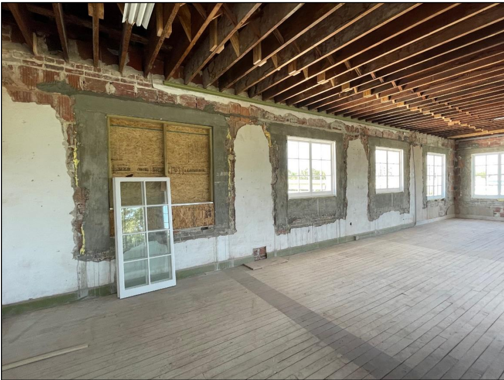
Figure 17: Interior photos showing concrete lintel reconstruction
