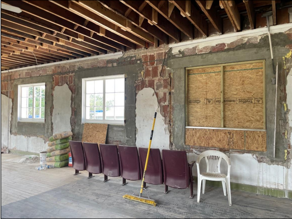
Figure 16: Concrete lintel reconstruction
