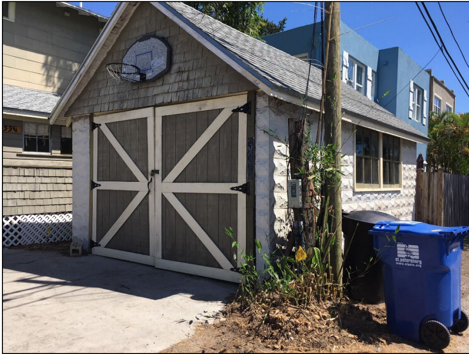
Figure 1: Garage building, which was converted into an accessory living space
