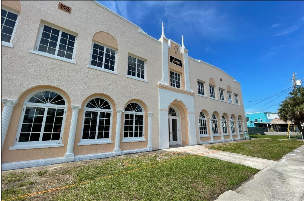
Figure 10: East side of front façade
