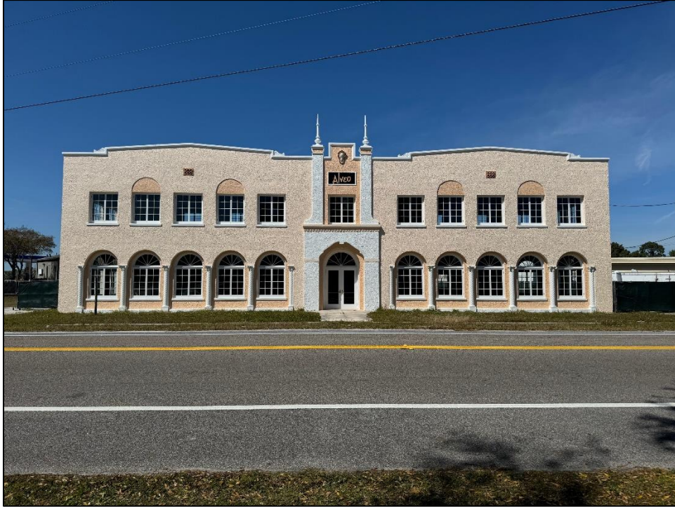
Figure 8: Front façade after reconstruction of porch columns, walls, and floors.
