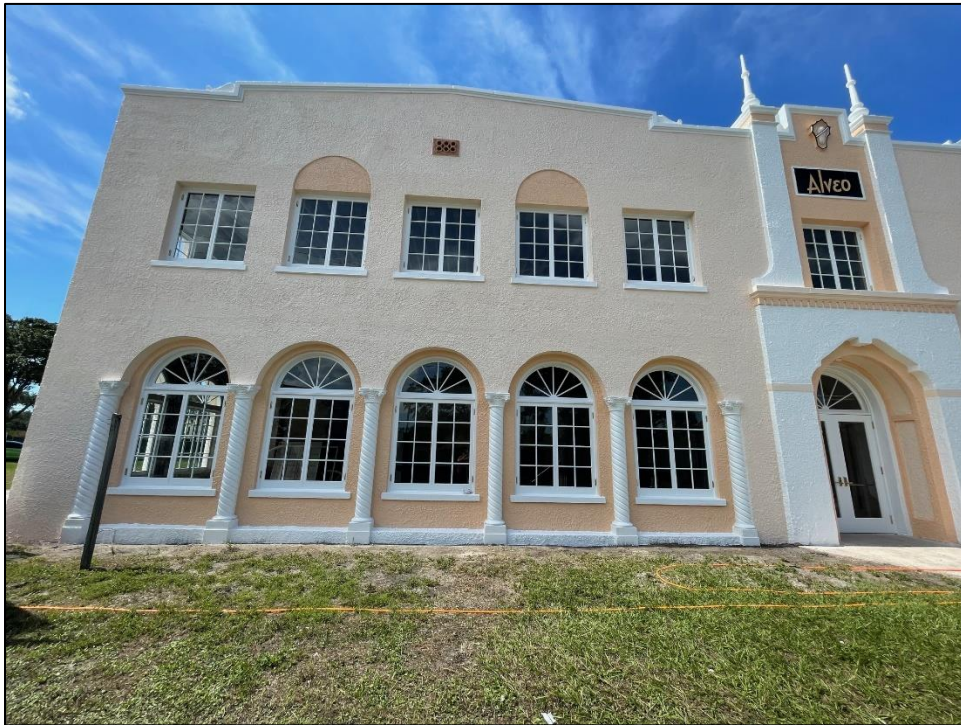
Figure 9: West side of front façade, after restoration
