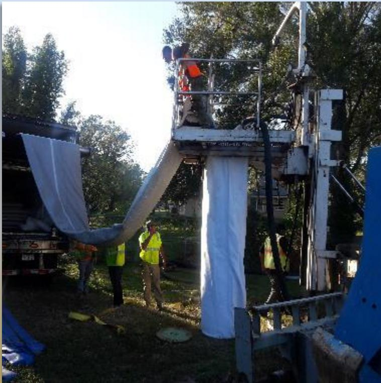
**Description:** Rehabilitate approximately 2.6 miles of large diameter sewer gravity pipelines.
