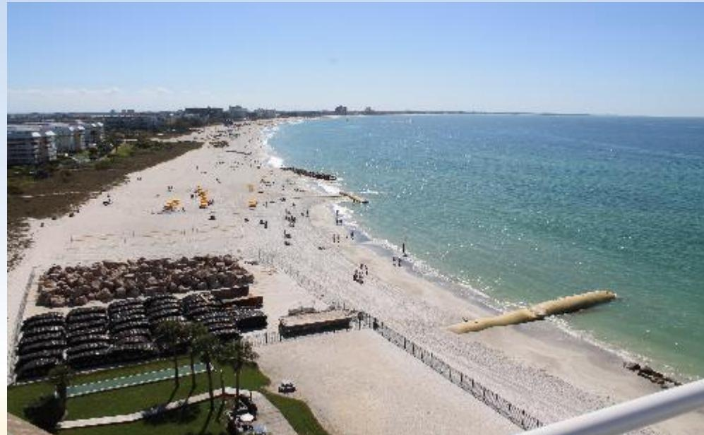
**Description:** Includes removal of 5 sand-filled geotextile bag t-groins and the installation of 4 rock t-groins.
