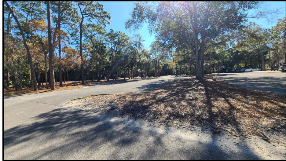
Inverness Hall parking area
