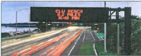
Highway Message Board
