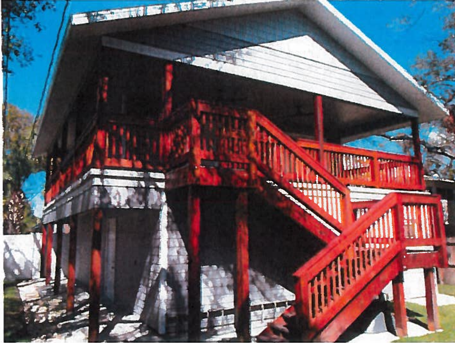
Photo 1: Frontal view (south) of new construction. Photo by Staff, 2018.
