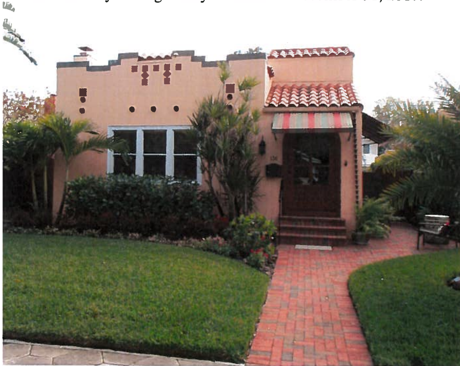
Keirn/Wehr Residence-post rehabilitation. Photo by Staff, 2018.
