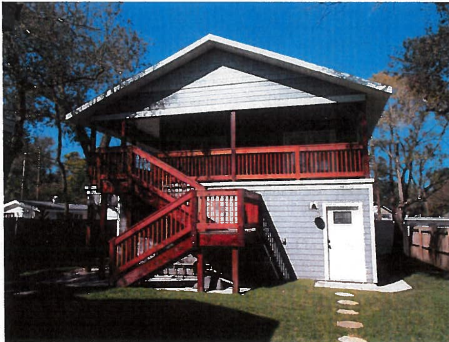
Matthews Property-frontal view of new garage/apartment. Photo by Staff, 2018.
