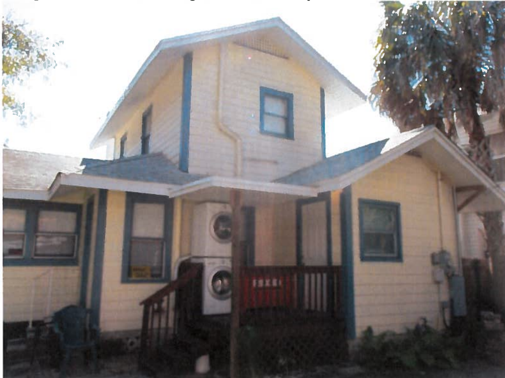
Photo 4: Historic main house reveals referenced gable roof forms, exterior clapboard siding, and 1/1 window configurations. Photo by Staff, 2018.
