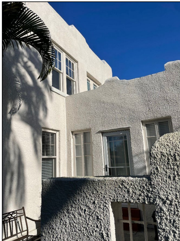
Figure 6: Side elevation, prior to construction
