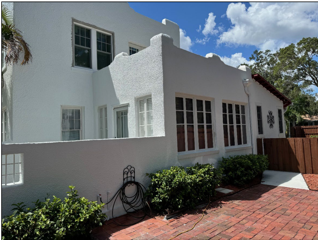
Figure 20: New side elevation, post construction
