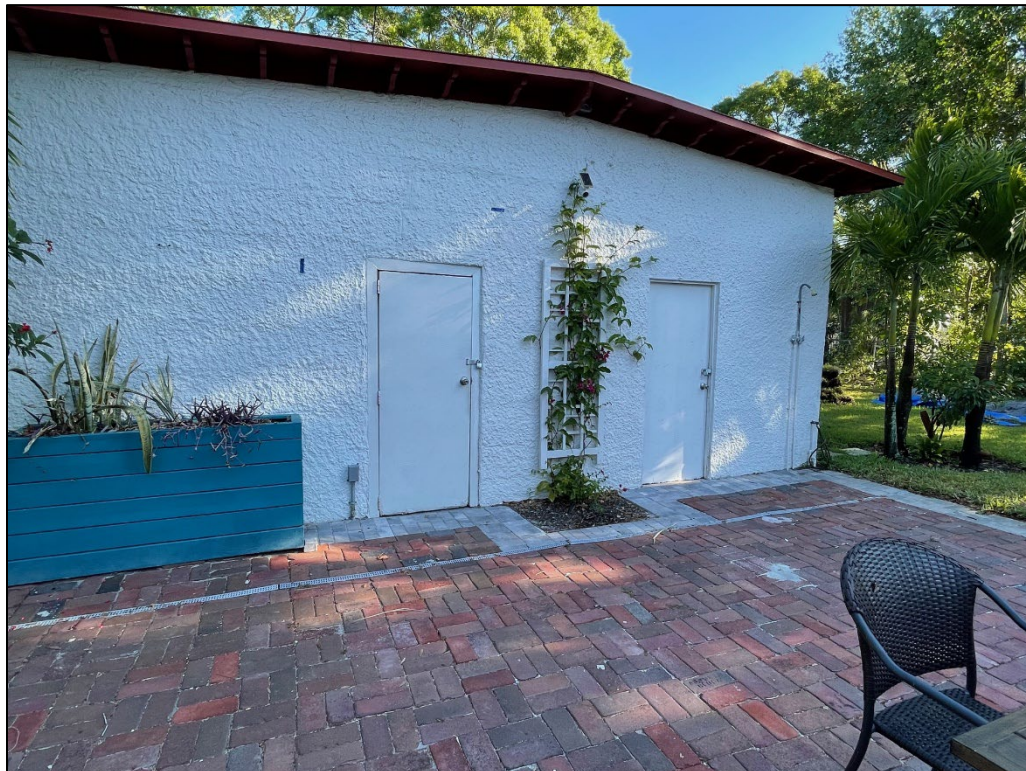
Figure 14: Garage wall cladding, prior to construction
