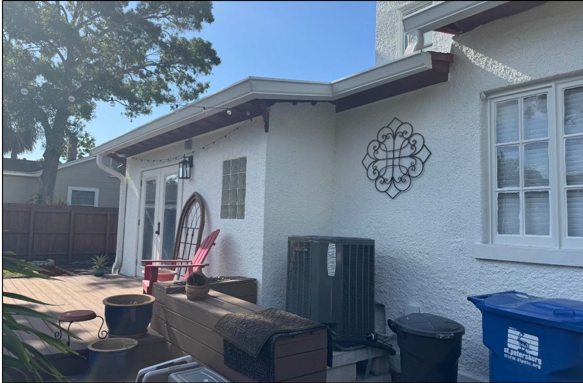
Figure 19: Rear elevation, post construction
