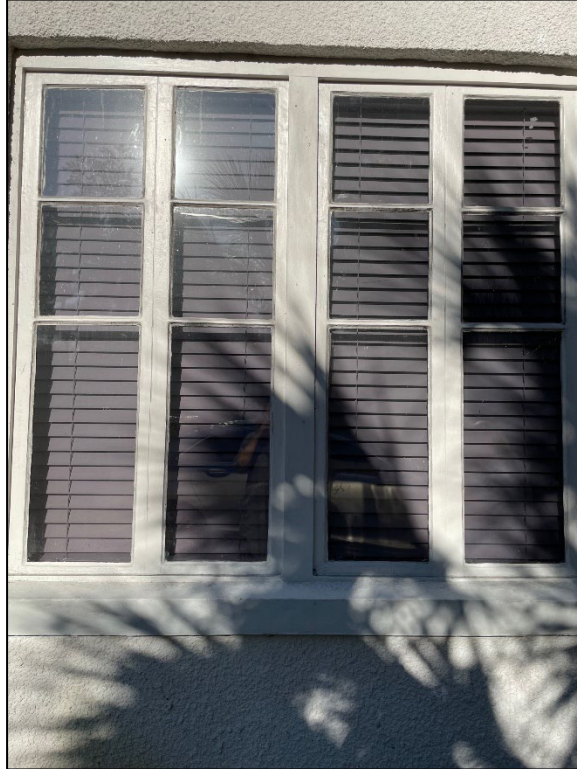
Figure 8: Window detail, prior to construction
