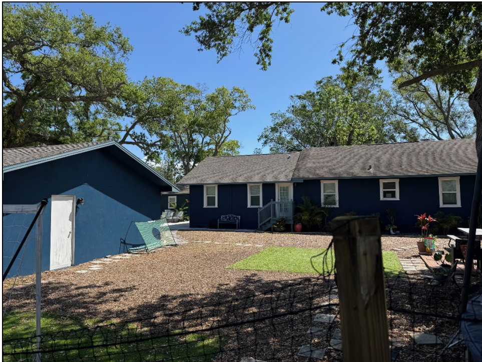
Figure 8: Side elevation, post construction
