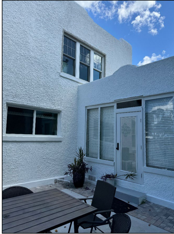
Figure 17: Side elevation, post construction
