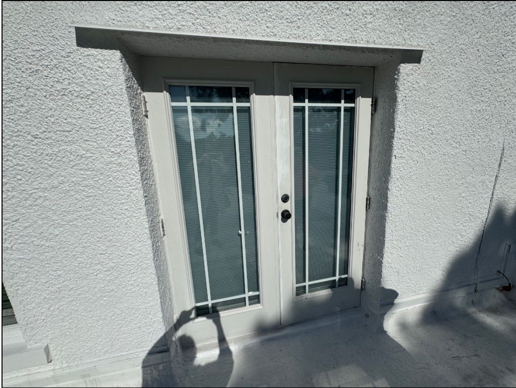
Figure 21: New French doors, post construction
