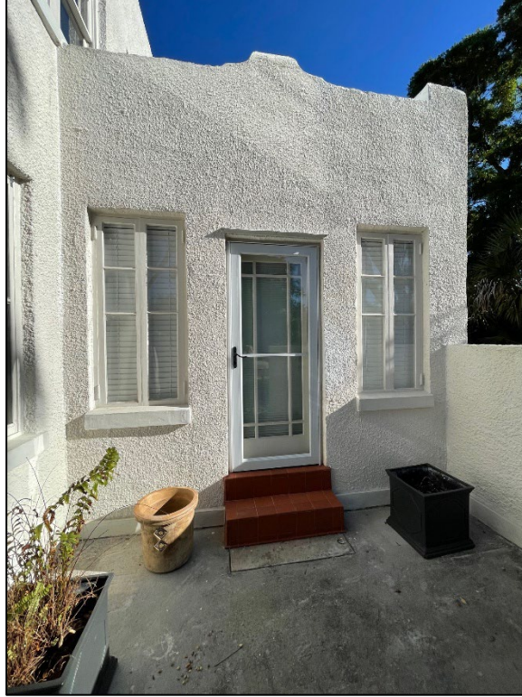
Figure 7: Side detail, prior to construction
