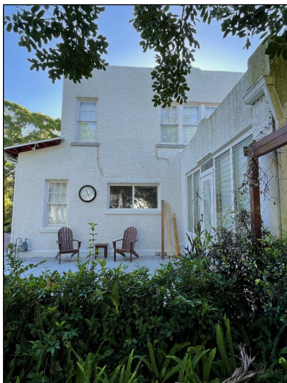
Figure 4: Side elevation, prior to construction
