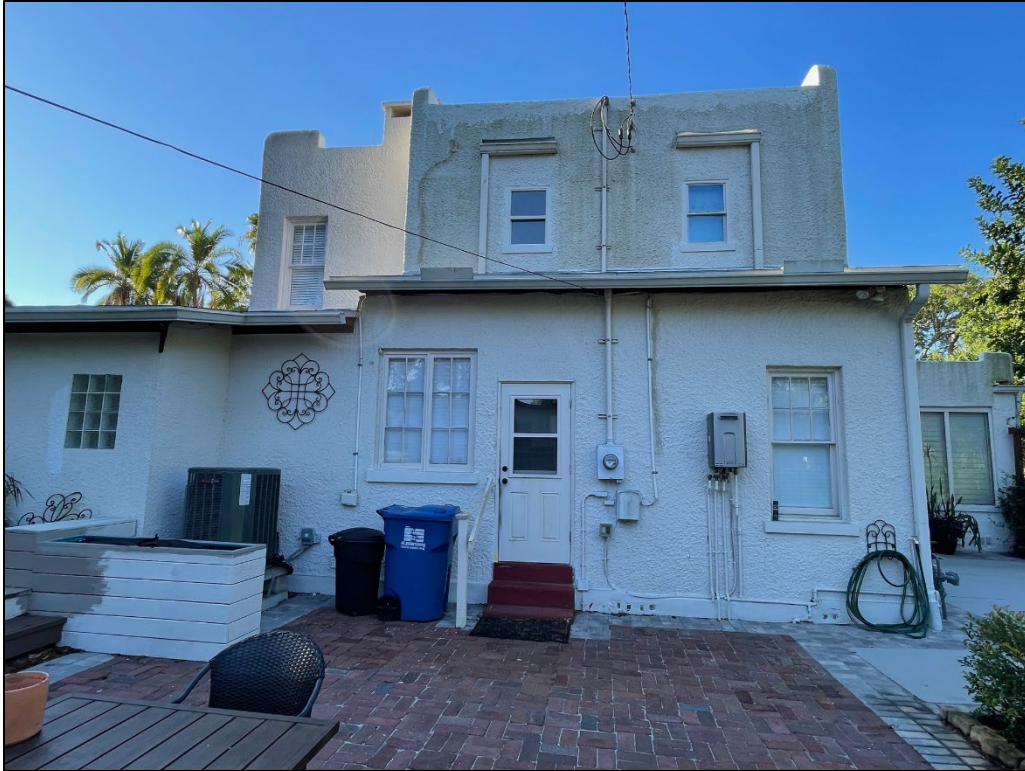
Figure 5: Rear elevation, prior to construction
