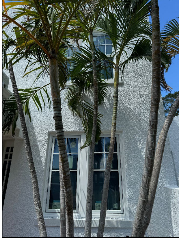
Figure 15: Exterior with new windows, post construction
