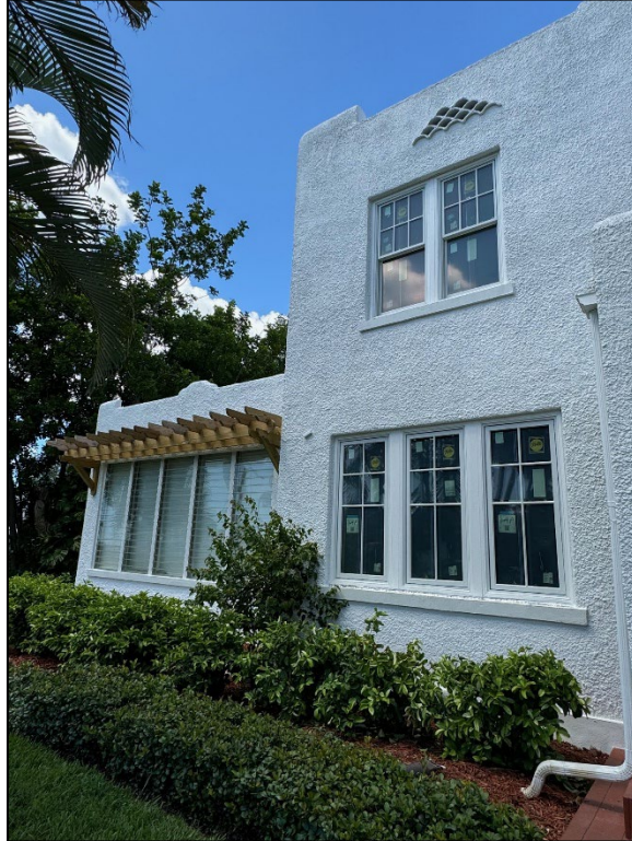
Figure 16: Front elevation, post construction
