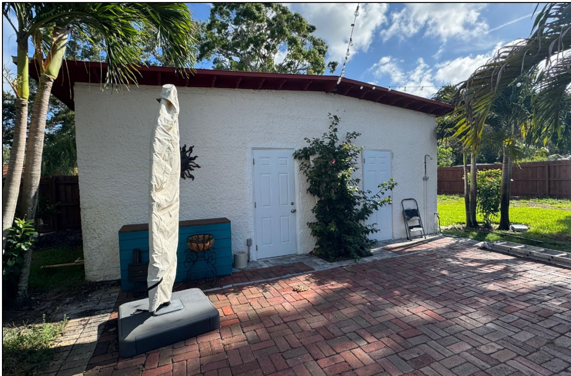
Figure 22: New garage cladding, post construction
