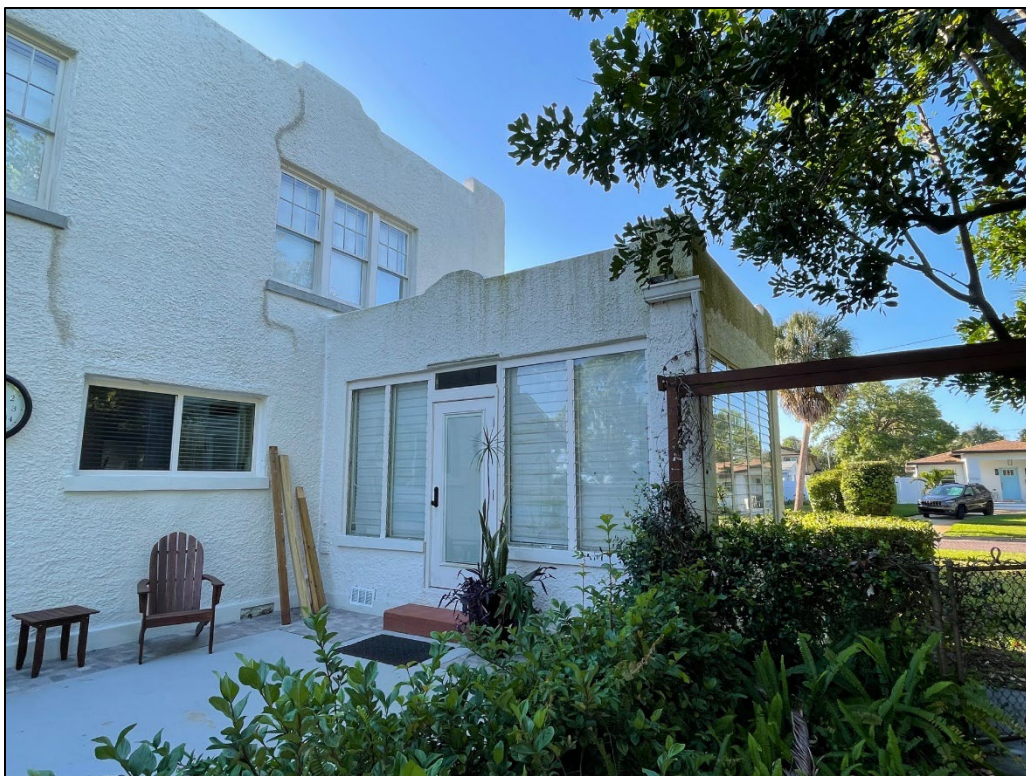
Figure 3: Side elevation, prior to construction
