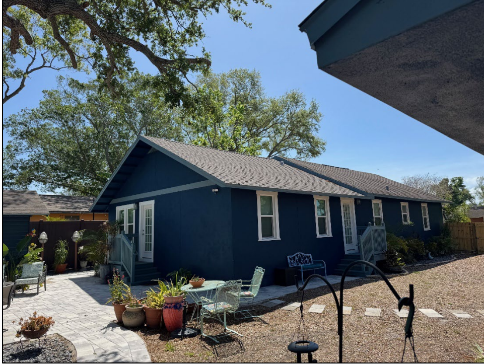
Figure 9: Rear elevation, post construction
