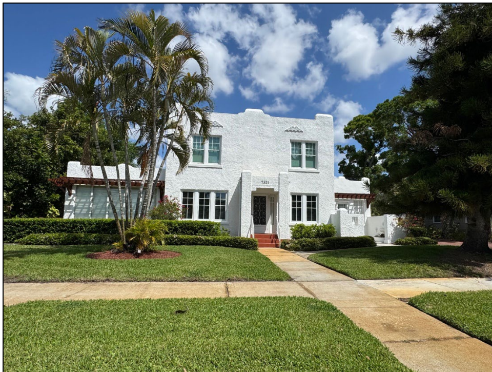
Figure 2: Front façade after rehabilitation.
