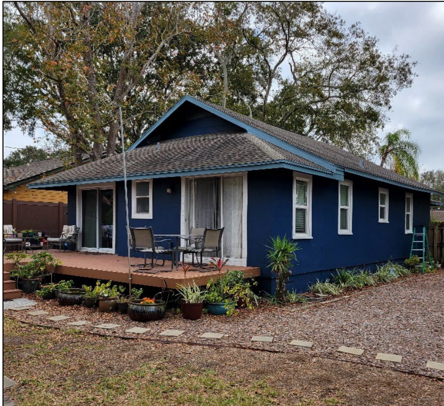
Figure 4: Rear elevation, prior to construction
