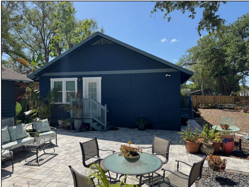
Figure 10: Rear elevation, post construction
