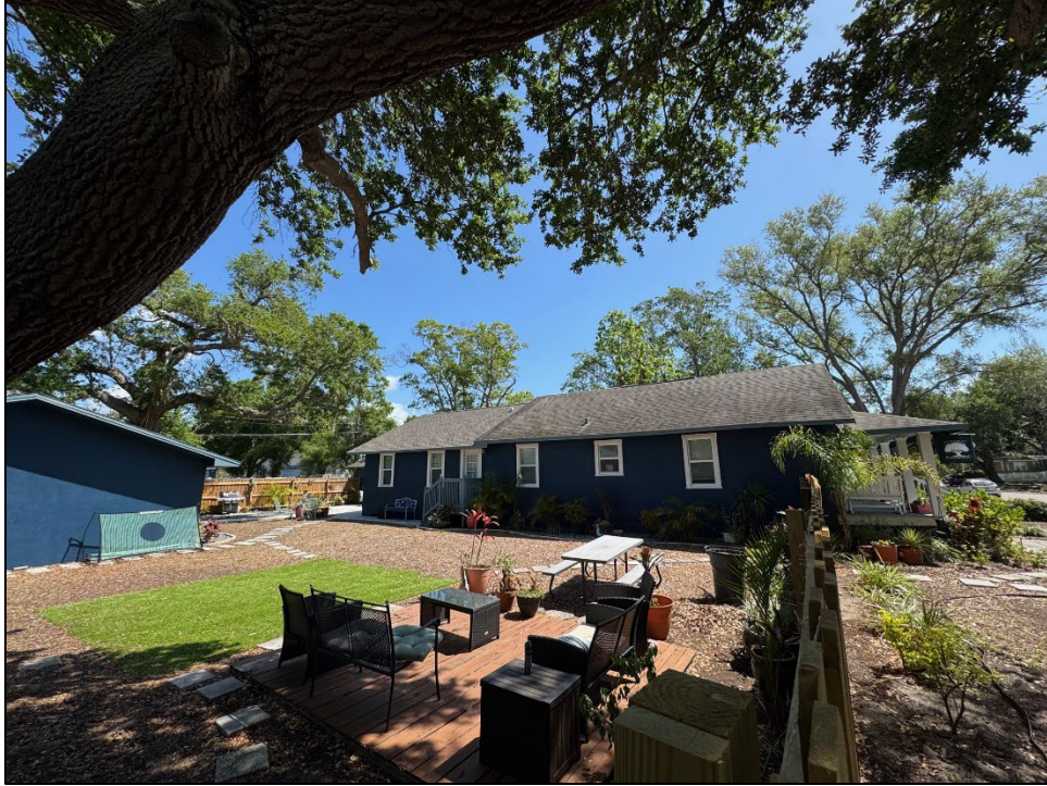
Figure 7: Side elevation, post construction
