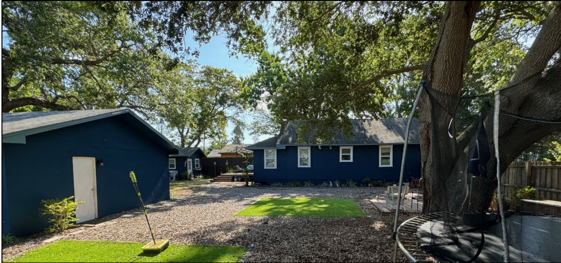
Figure 3: Side elevation, prior to construction
