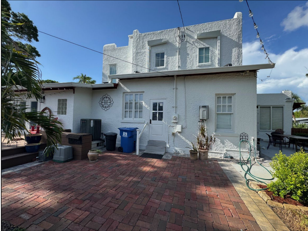
Figure 18: Rear elevation, post construction
