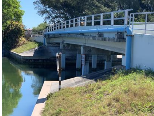
Sands Point Drive/13 th St Bridge Water Line
