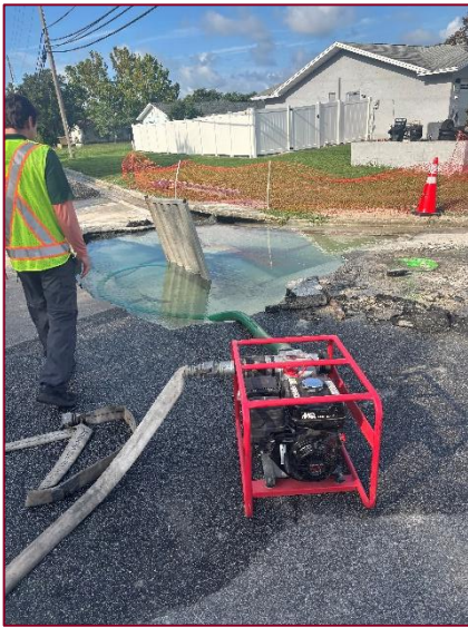
Figure 3 - Public Works Emergency Water Main Repair
