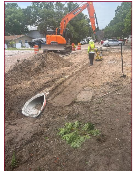
Figure 4 - Public Works Storm Drain Installation
