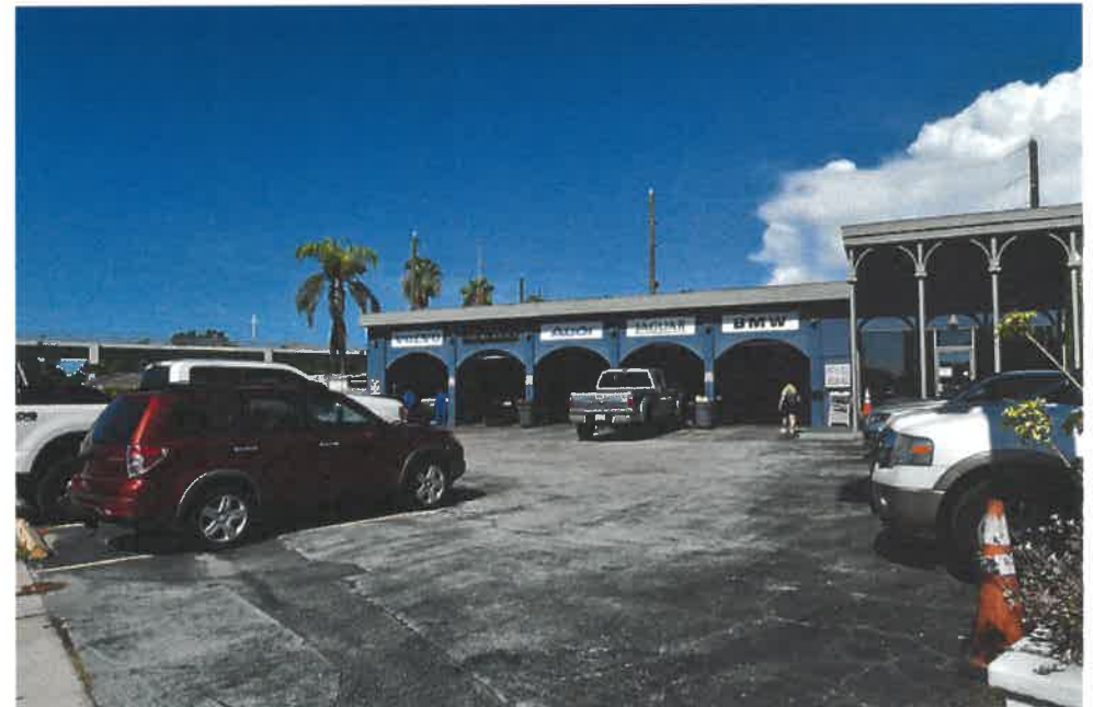
Pasadena Ave Facing West
