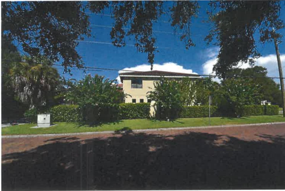
71 st St S ROW - Facing West Existing Single Family Homes NT-3 Min. Setback Street Side Yard = 15 Ft
