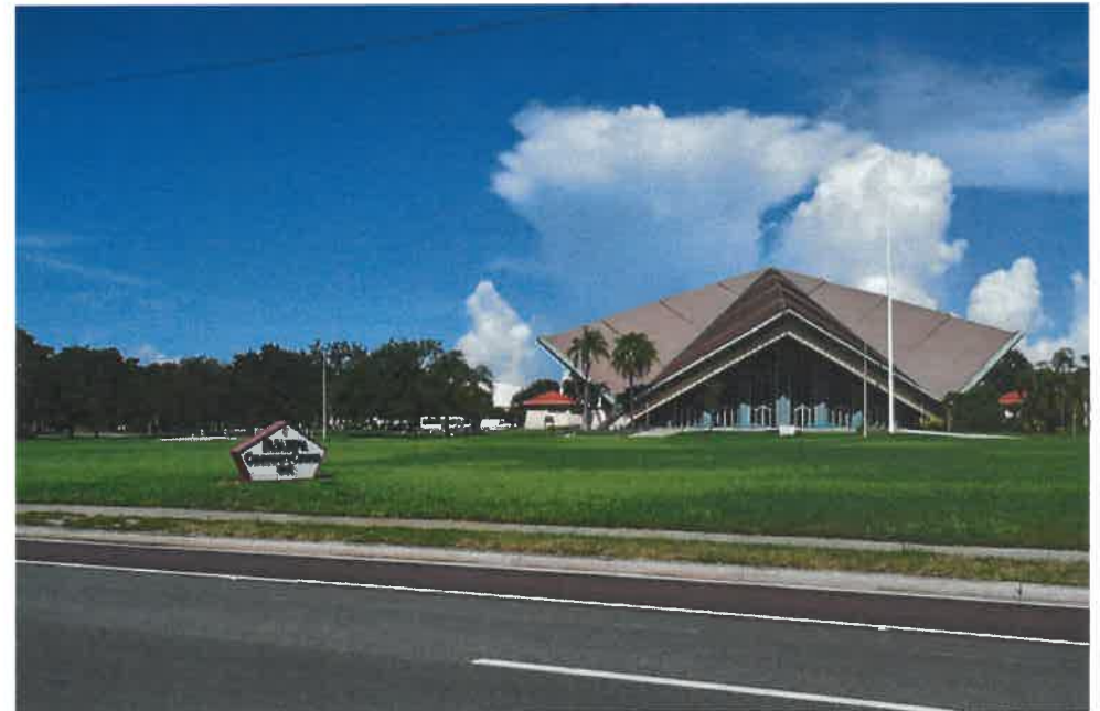
Pasadena Ave Facing West
