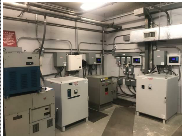
Photo #8 Vault – Interior – East Room – Representative Overview
