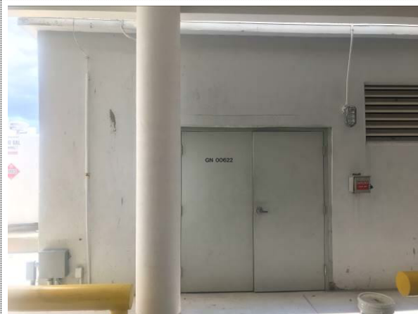
Photo #1 Vault – Exterior – Representative Overview
