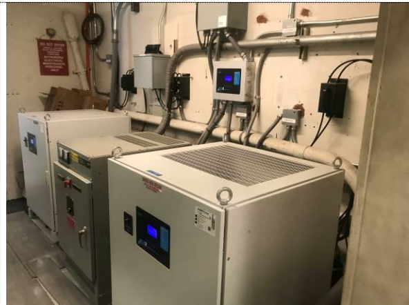
Photo #9 Vault – Interior – Center Room – Representative Overview
