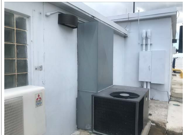
Photo #4 Vault – Exterior – Representative Overview
