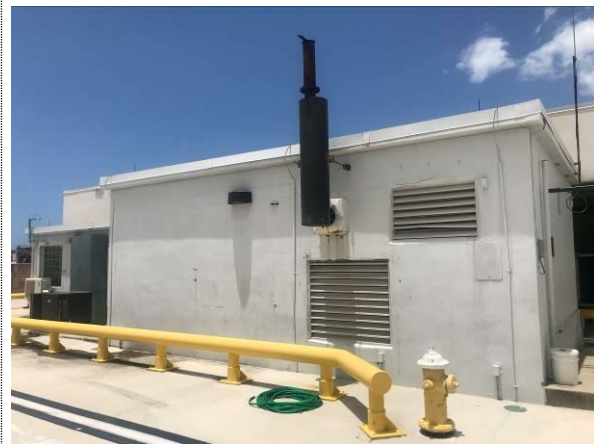
Photo #3 Vault – Exterior – Representative Overview
