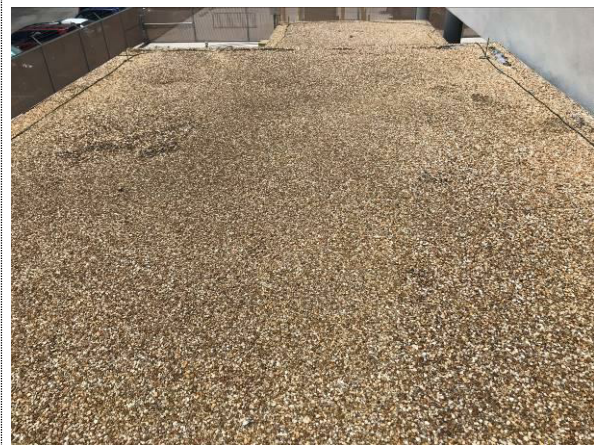
Photo #5 Vault – Roof – Representative Overview
