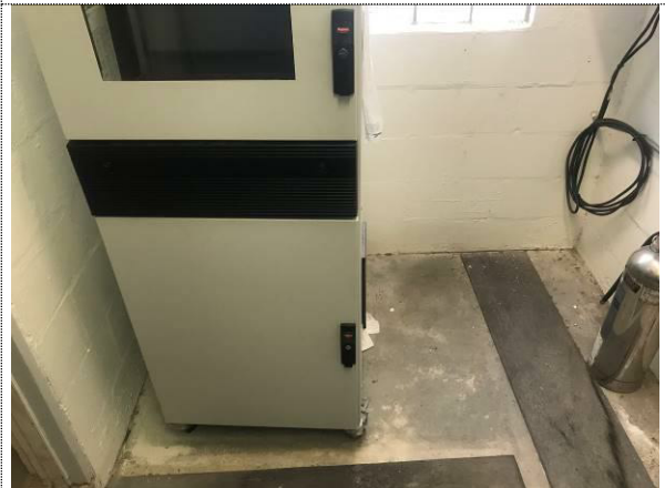
Photo #12 Vault – Interior – West Room – Representative Overview
