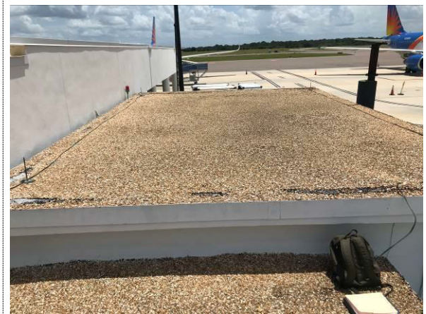
Photo #6 Vault – Roof – Representative Overview
