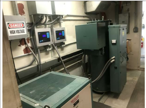
Photo #10 Vault – Interior – Center Room – Representative Overview
