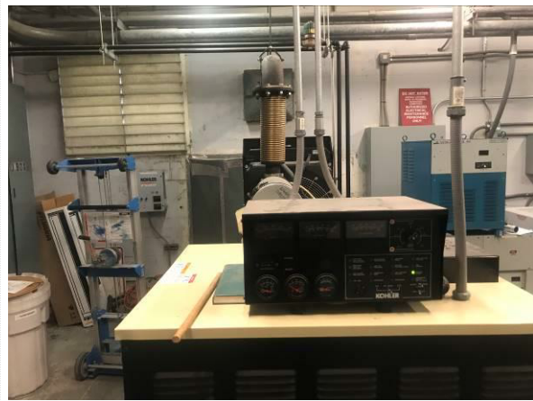
Photo #7 Vault – Interior – East Room – Representative Overview
