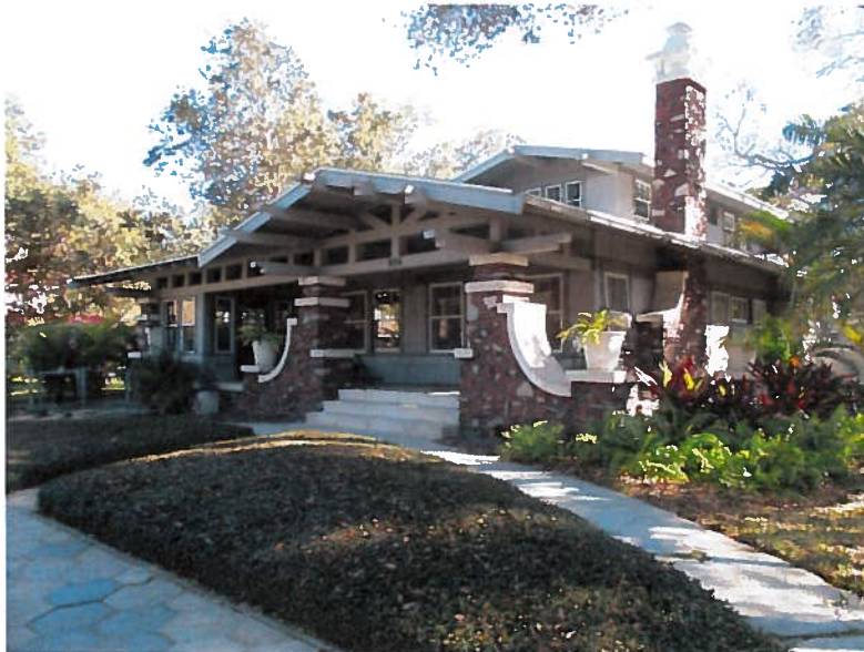
Reid/Winters Residence-post rehabilitation. Photo by Staff, 2016.
