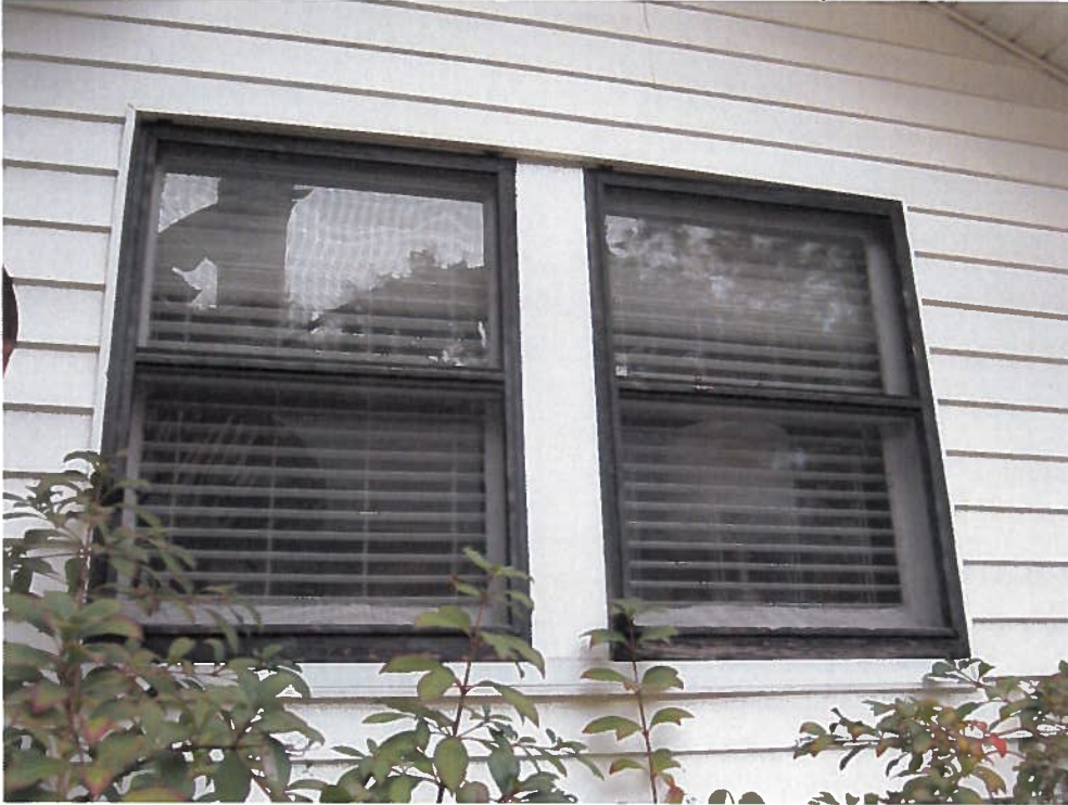
Photo 6: View historic double-hung window sets. Photo by Staff, 2014.
