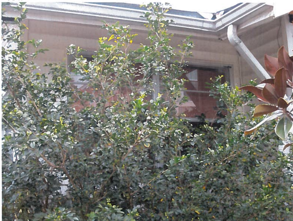
Photo 5: View non-historic, pre-construction aluminum window sets. Photo by Staff, 2014.
