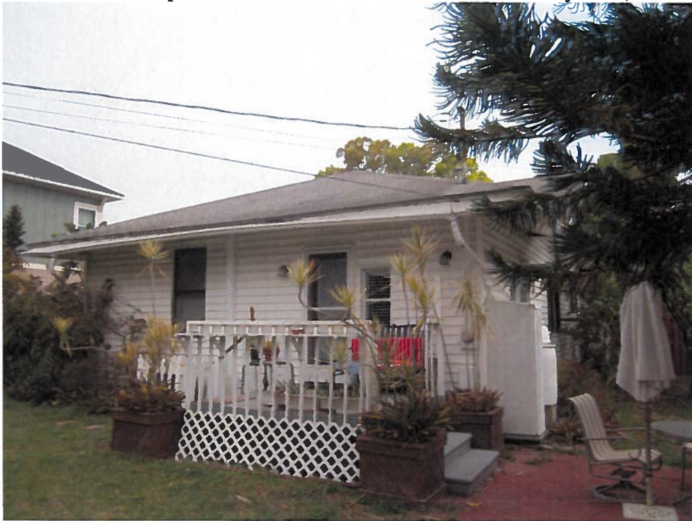
Photo 4: View of pre-construction rear/side elevation. Photo by Staff, 2014.
