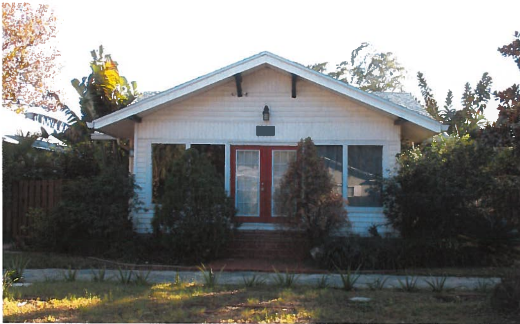
Rosenberg Residence-post rehabilitation. Photo by Staff, 2017.
