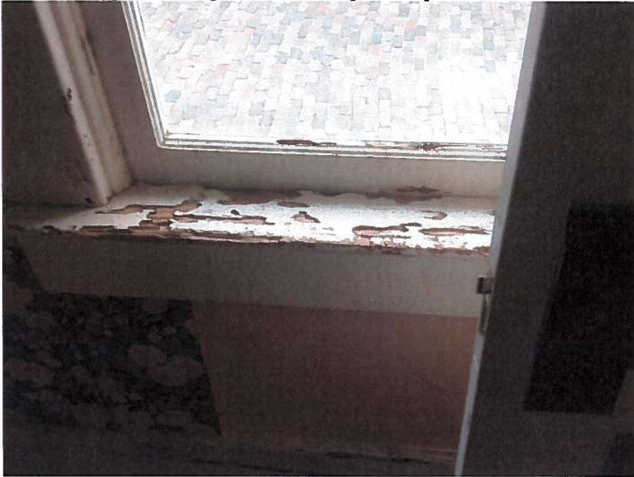
Photos 5a, b: Active rehabilitation of interior. Photo by Staff, 2016.
