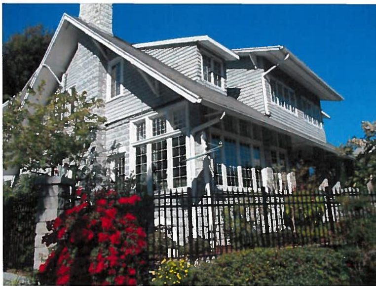
Sadler Residence-post rehabilitation. Photo by Staff, 2017.
