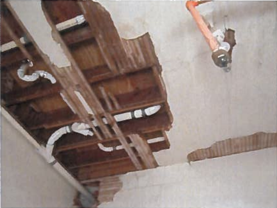
Photo 5: Typical plumbing upgrade showing active work. Photo by Staff, 2013.
