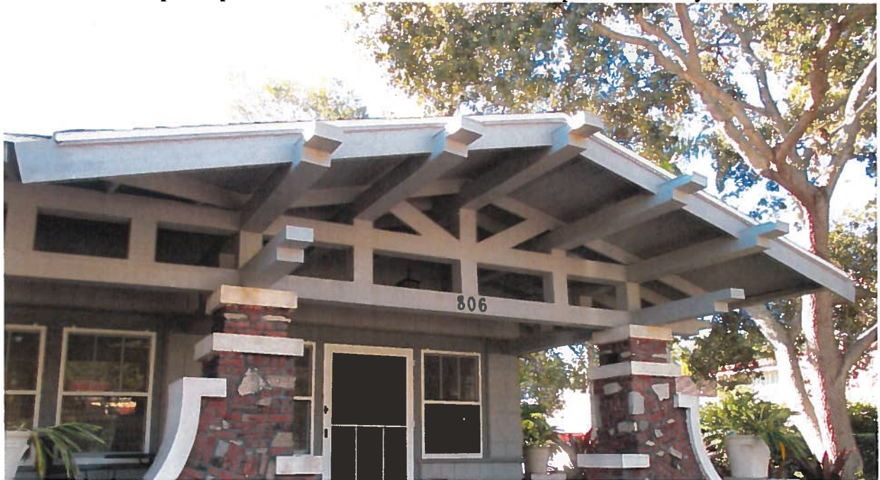
Photo 5: Close-up of repaired roof beams/structure at frontal porch. Photo by Staff, 2017.
