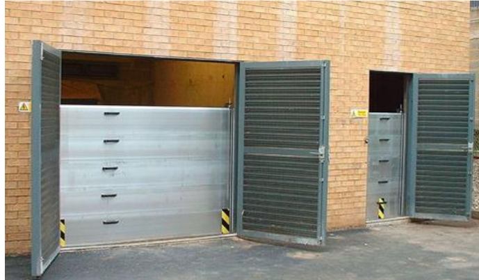
Figure 12: Deployable Dry Floodproofing Retrofit
