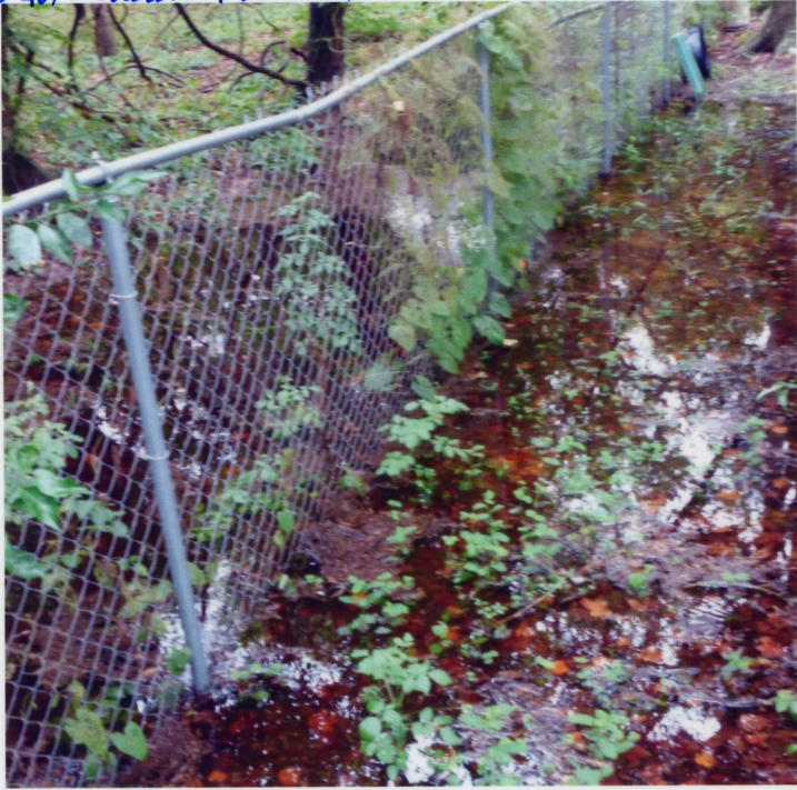
2204 Lawton looking east down property line
