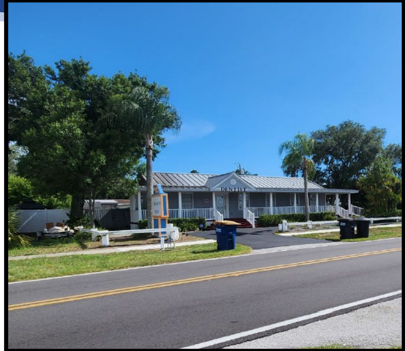
Office use to the West
