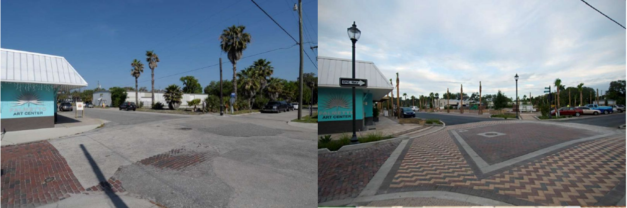
Figure 6.5.1: Where would you rather shop/dine? (5th Street in Palmetto, FL before and after revitalization using green infrastructure – Applied Sciences, Inc.)
