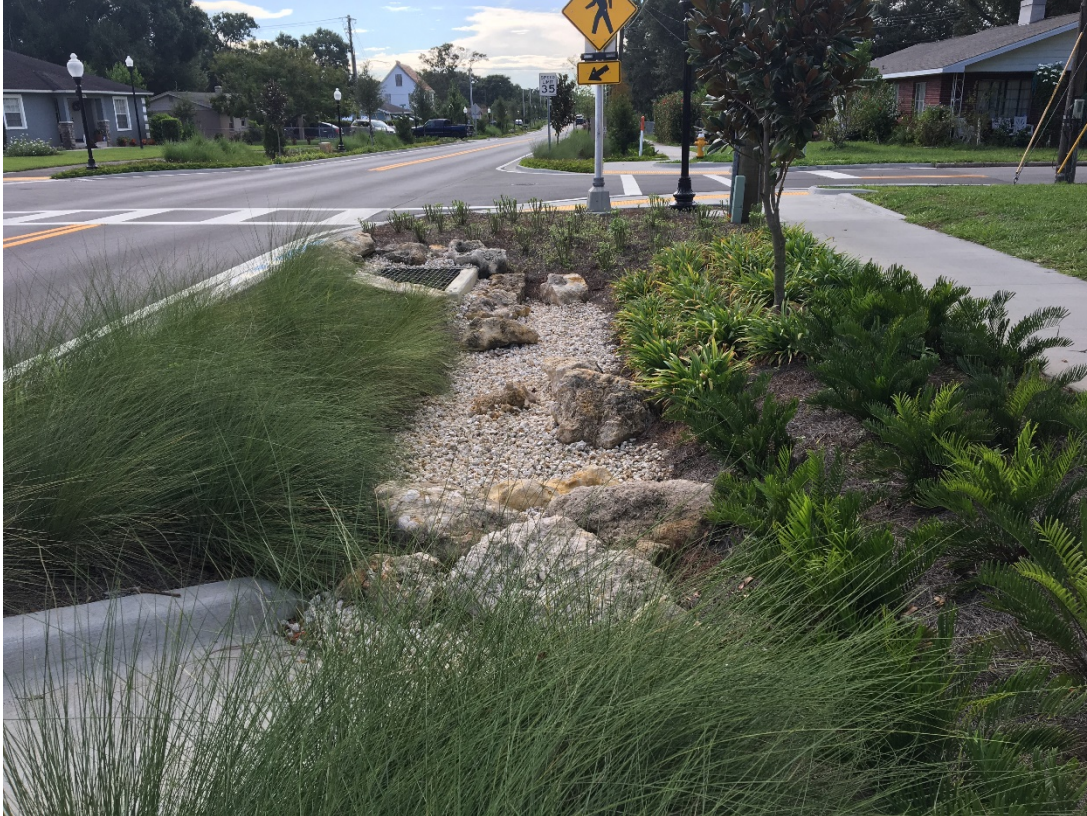
PK Avenue bioswale – Auburndale, FL
