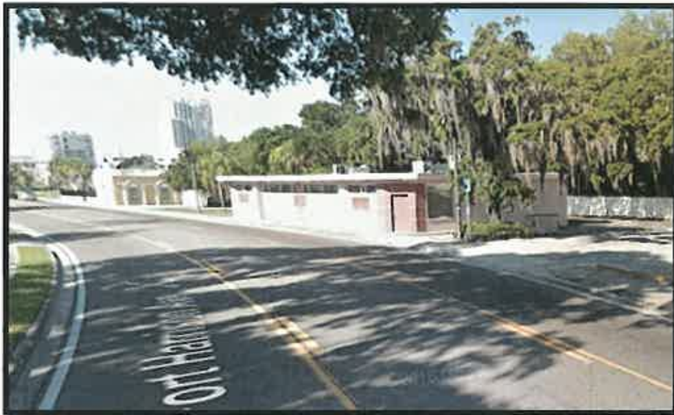
Northside of building
