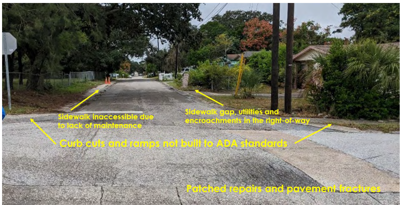
Figure 8 Inadequate Transportation Infrastructure: Pavement and Accessibility
