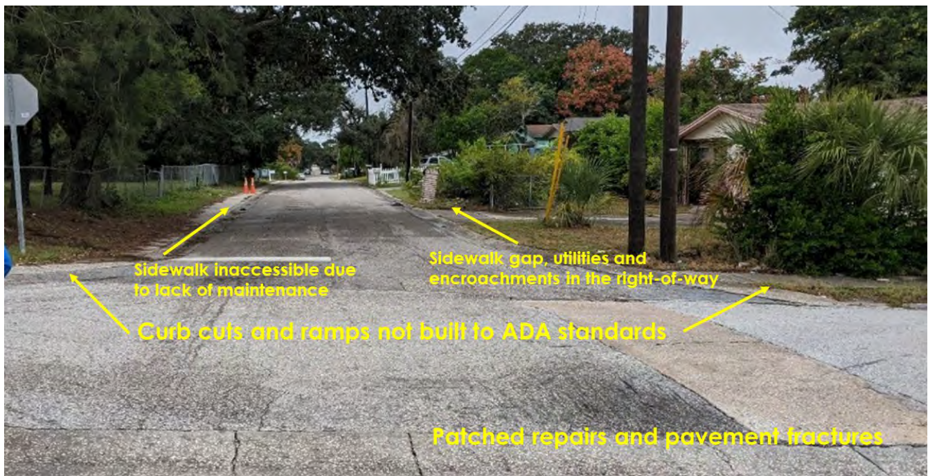
Figure 8 Inadequate Transportation Infrastructure: Pavement and Accessibility
