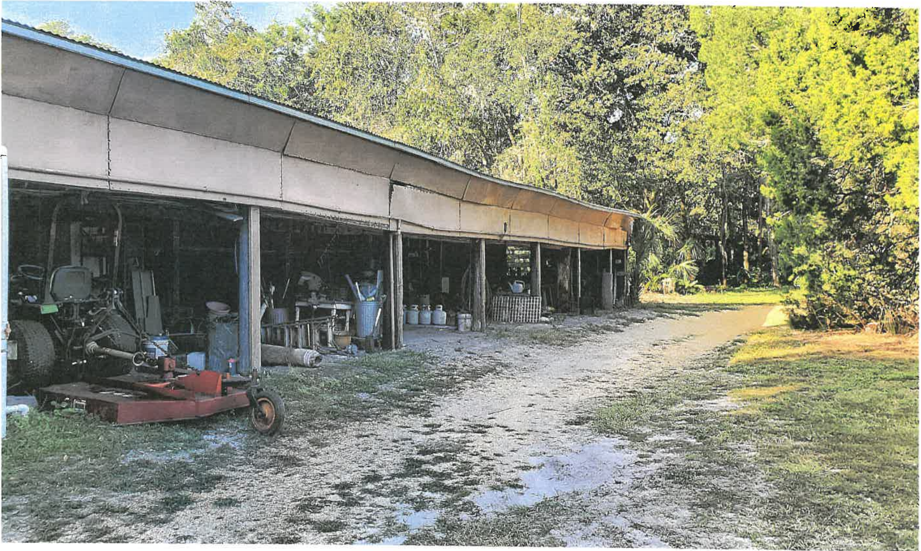
Existing shed structure located South of the home
