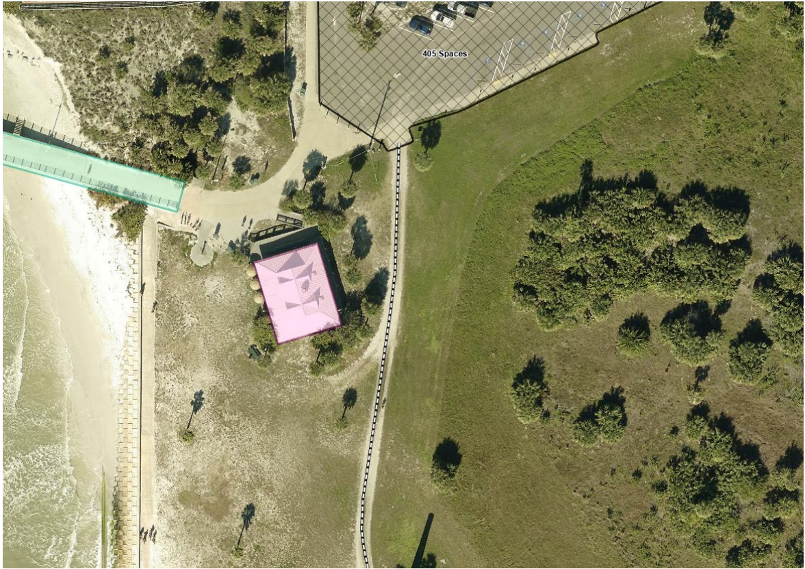
3. The Gulf Pier snack bar/bait shop, a 1,200 square foot building that includes restroom facilities to be cleaned by the concessionaire. Located at 27.613000, -82.736650.
