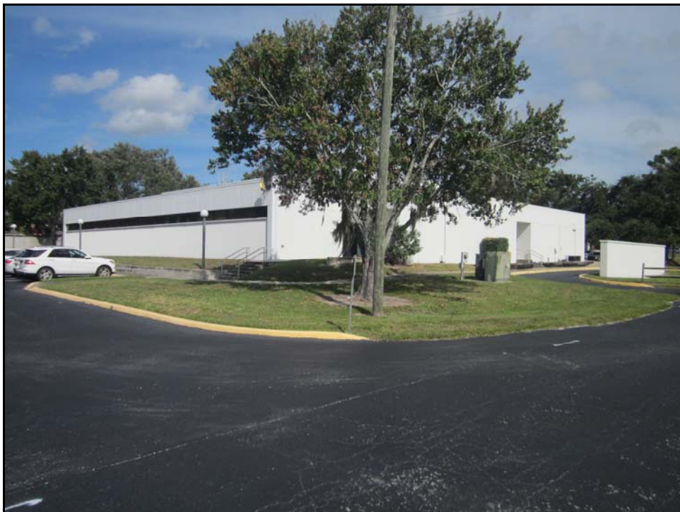
Photo 18: Looking northeasterly at south and west elevation of the Government Services Building.
