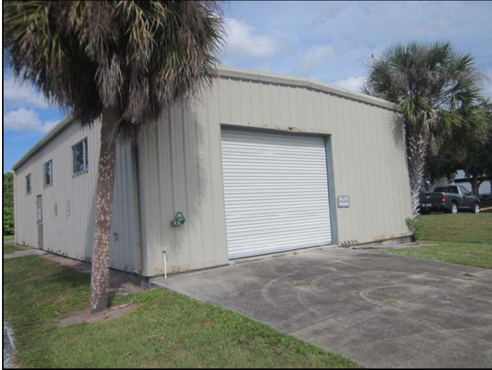
Photo 17: Looking northeasterly at south and west elevation of metal storage building.
