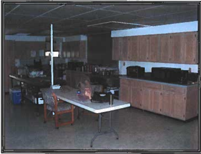
Kitchen in the Fellowship Hall/Office Building
