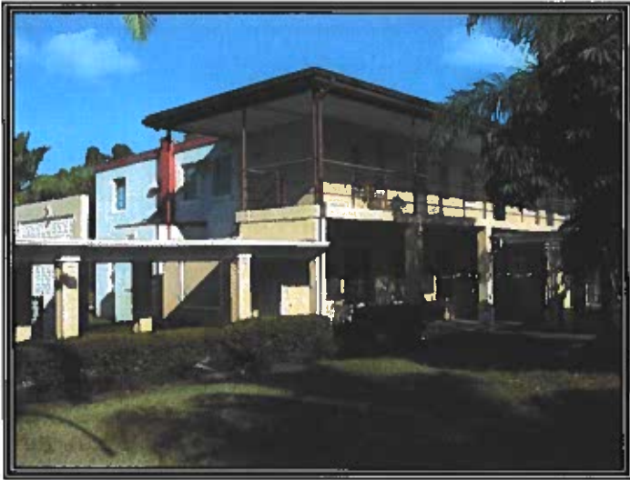
Looking Northwest at the Southerly End of the Education Building
