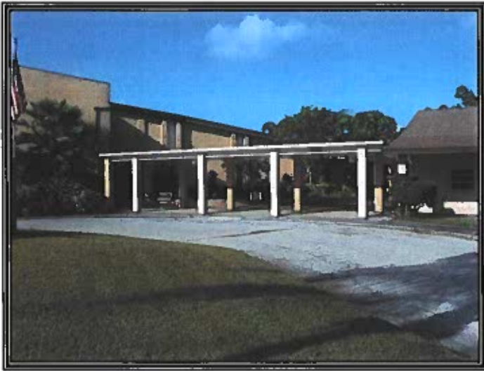
Front Entrance Drive Looking Toward the North Elevation of the Sanctuary
