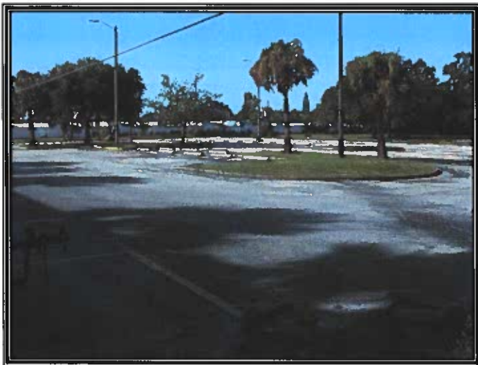
Looking Southwest From Behind the Education Building at the Rear Parking Lot and Site
