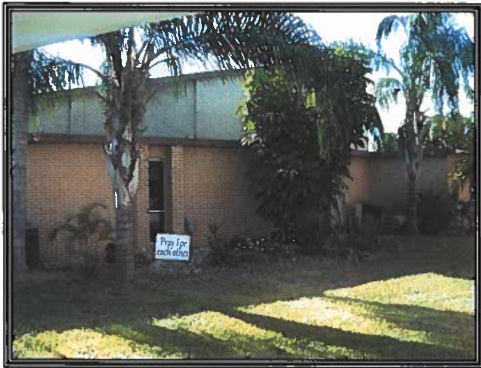
Rear Elevation of the Sanctuary
