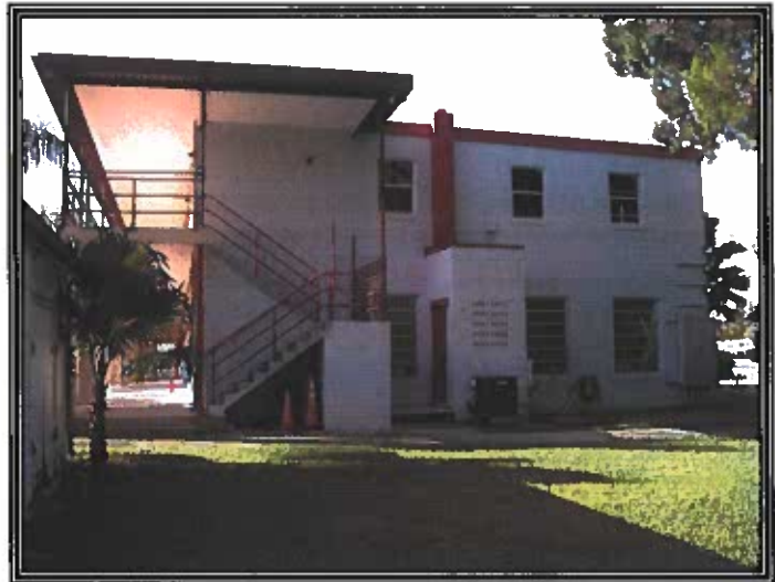
North End of the Education Building
