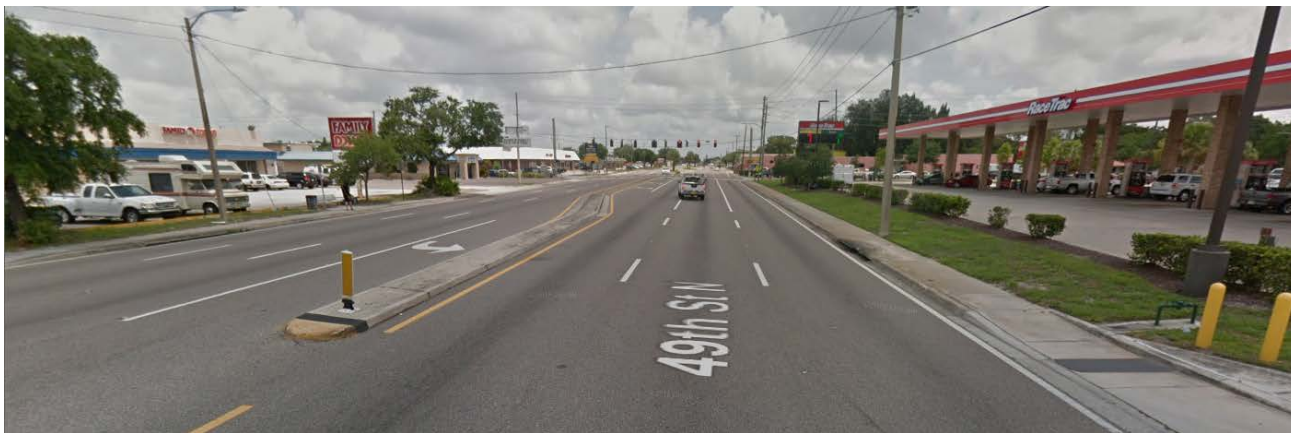
No bicycle facilities
