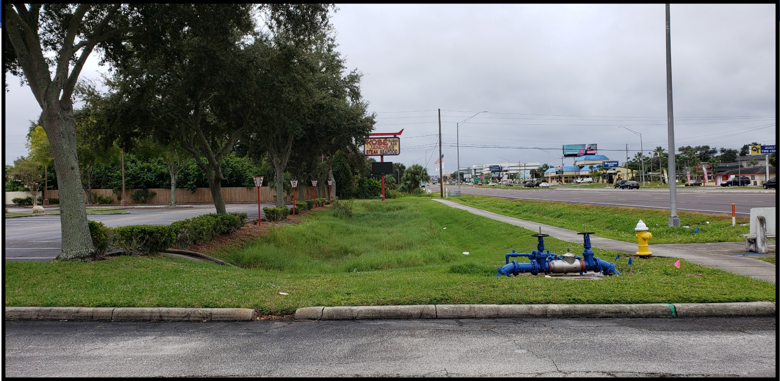
Looking south along US Highway 19
