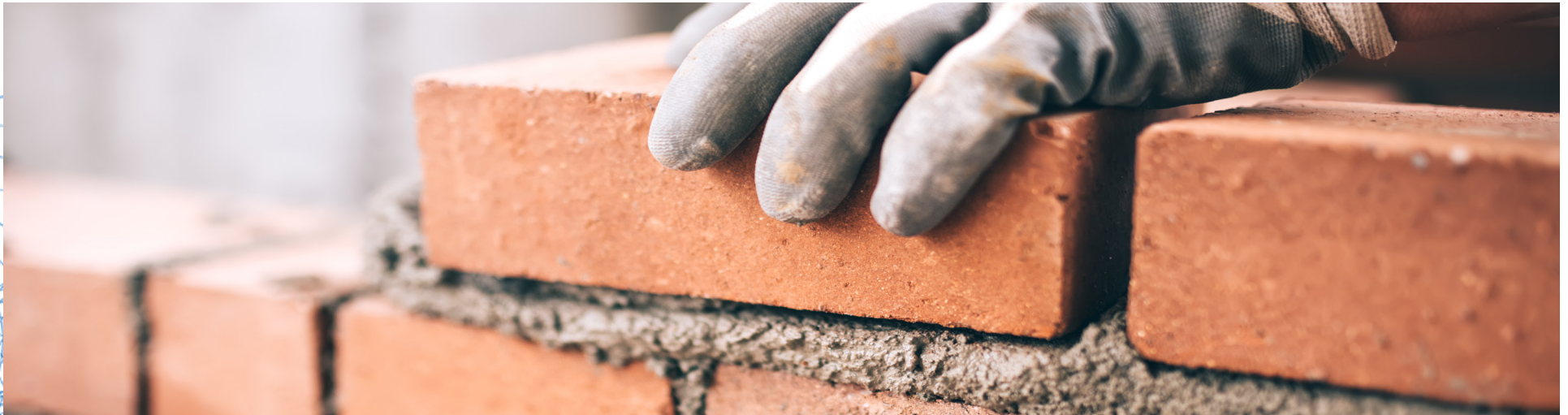
Brick laying at a construction site
