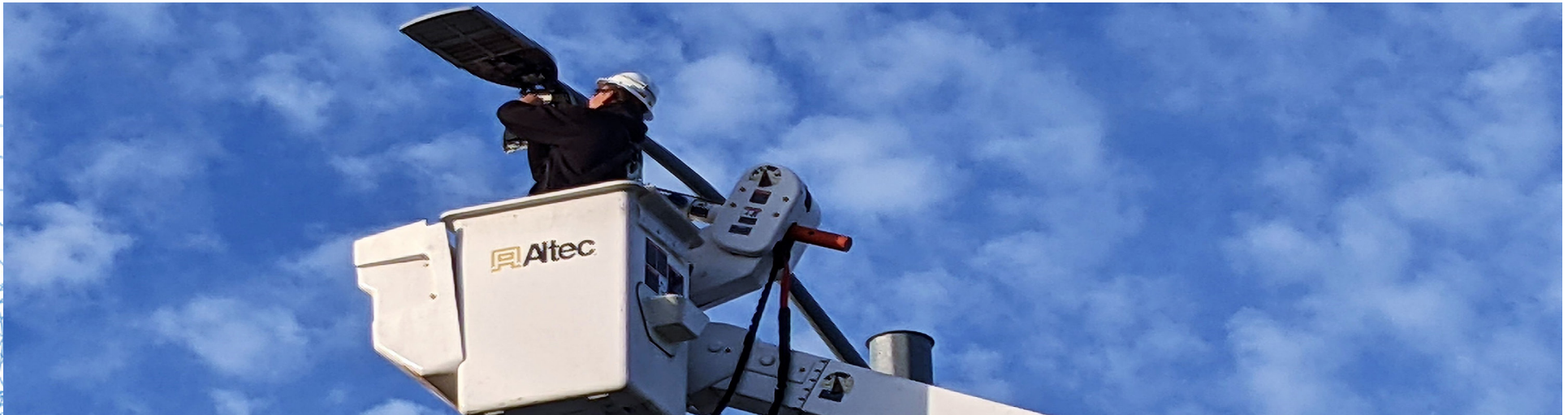
LED Street Light Installation
