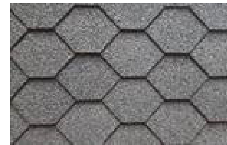
Asphalt shingle, diamond or hexagonal
