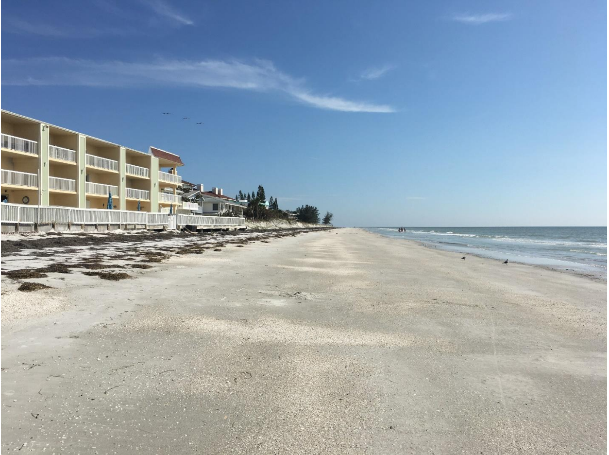
Figure 2-1: Post Storm view of berm erosion and water line pushed up to near the shorefront infrastructure just south of R-84 on Sand Key.
