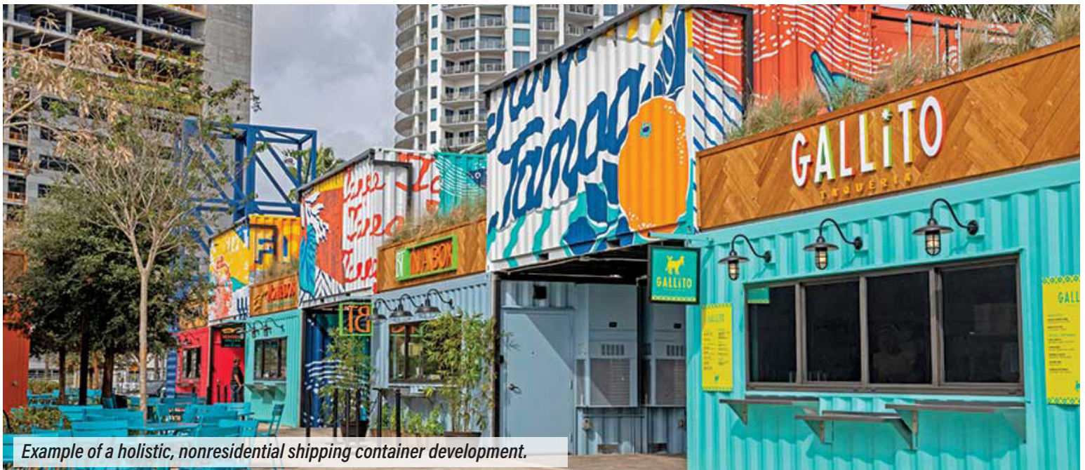
Example of a mixed-use structure constructed of shipping containers.
