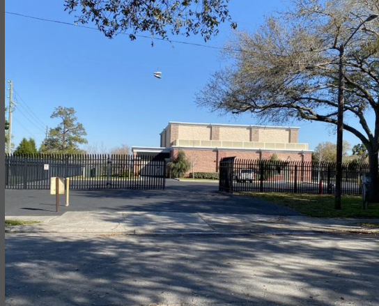
b. Water Treatment Facility (south)
