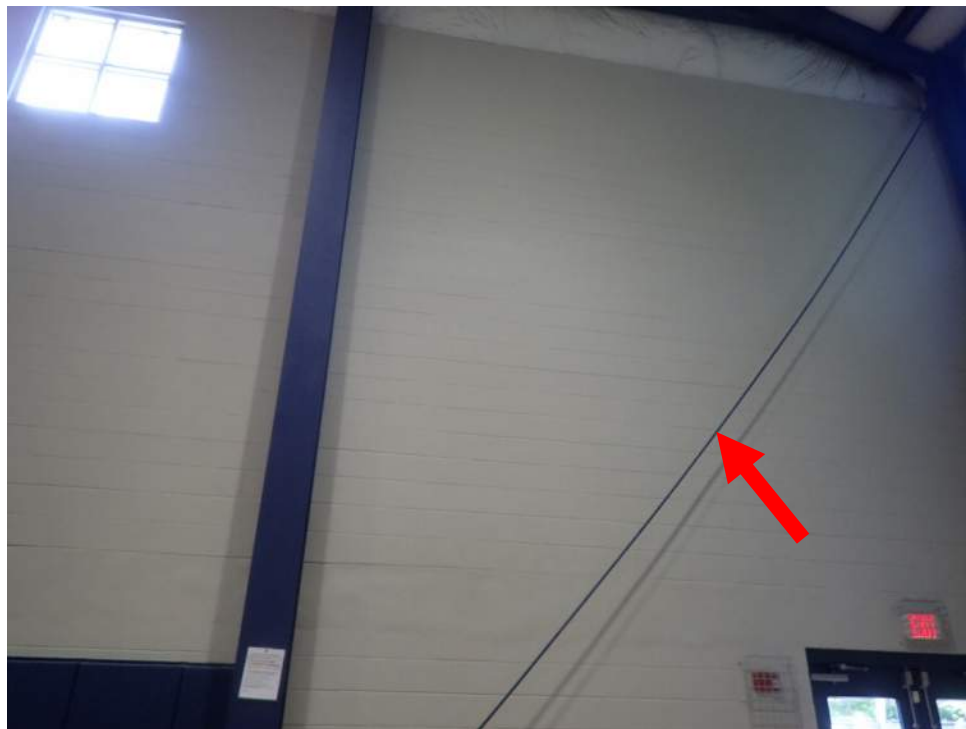
Photograph 8 – Loose X Bracing between Rigid Frames
