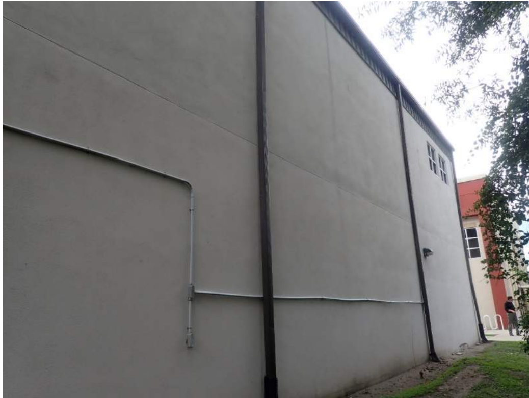
Photograph 5 – Partial East Elevation (Right side)
