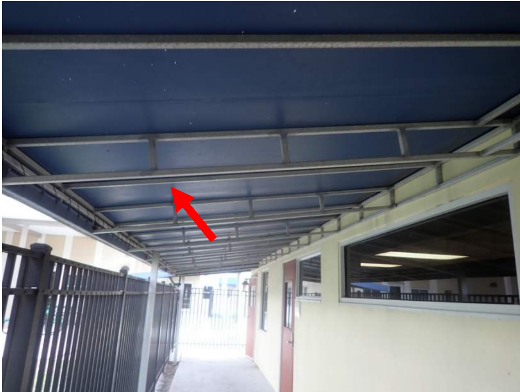
Photograph 11 – Canopy Attached To Exterior Walls
