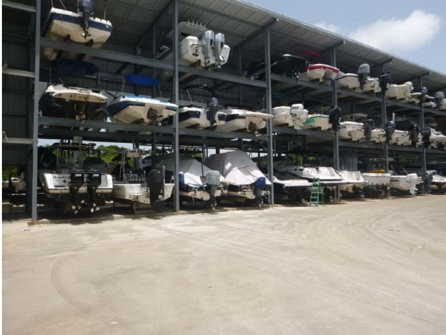
VIEW OF SUBJECT PARCEL FACING NORTHWESTERLY FROM WITHIN THE MARINA DEVELOPMENT Note: The subject is the land under the building
