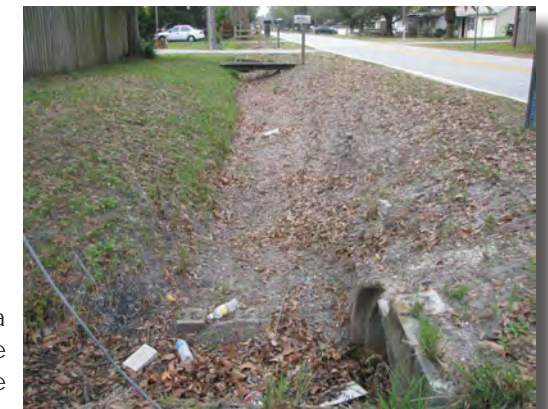
Existing Area Drainage Infrastructure
