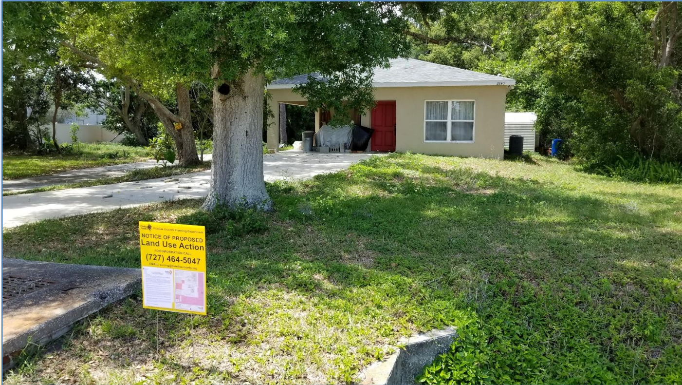
Existing Single Family Home
