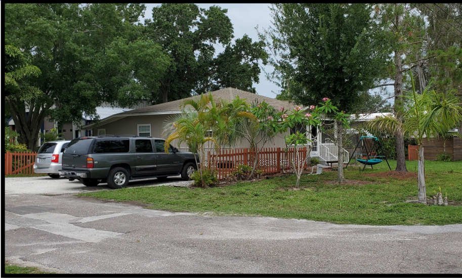
Looking at house to the north
