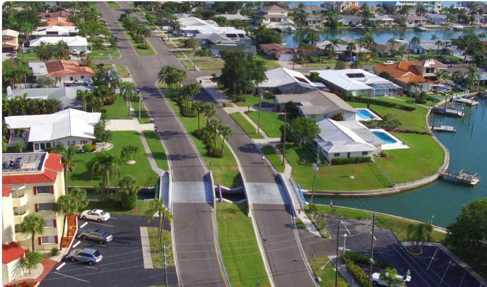
Island Estates Bridge: after replacements
