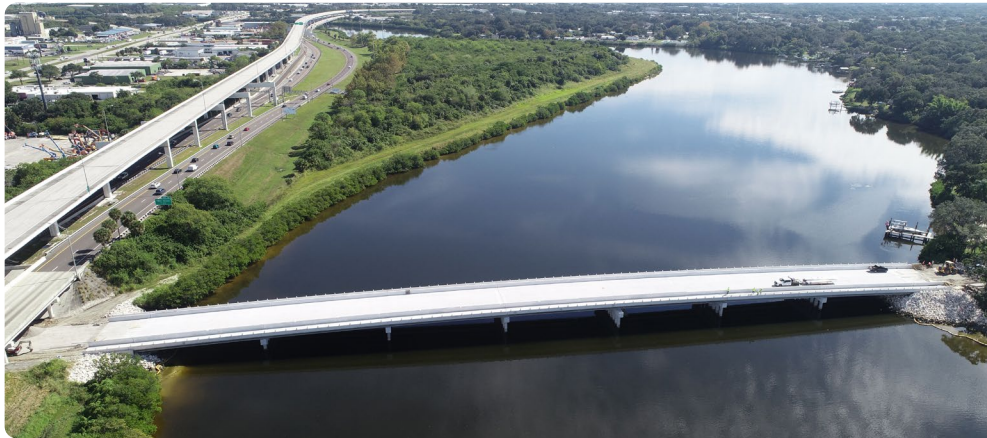
Maydell Drive Bridge: after construction
