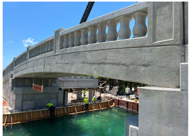
Bimini Drive Bridge: under construction
