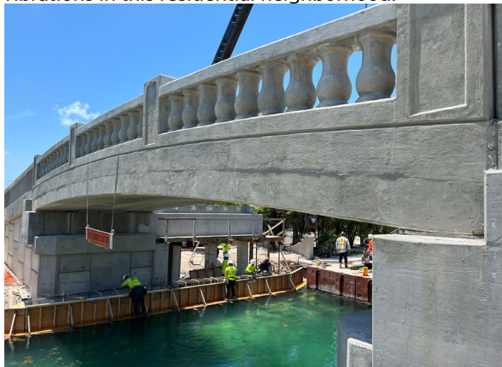
Bimini Drive Bridge: under construction
