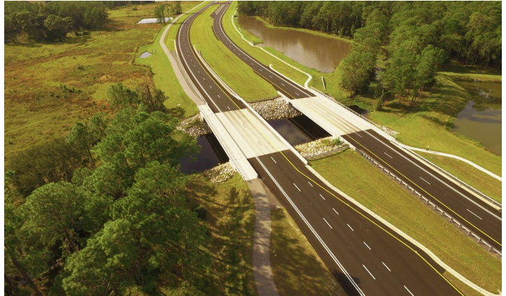
SR 56: after construction
