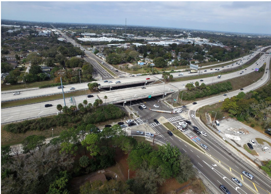
TBNext Segment 2: current conditions
