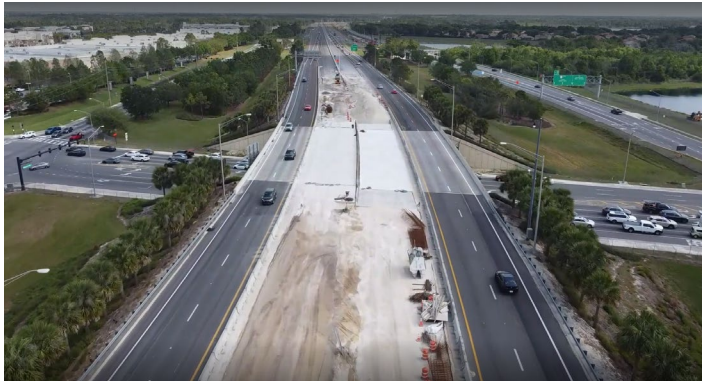
SR 429 Widening: under construction
