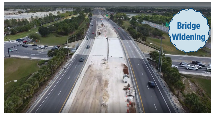
SR 429 Widening: under construction
