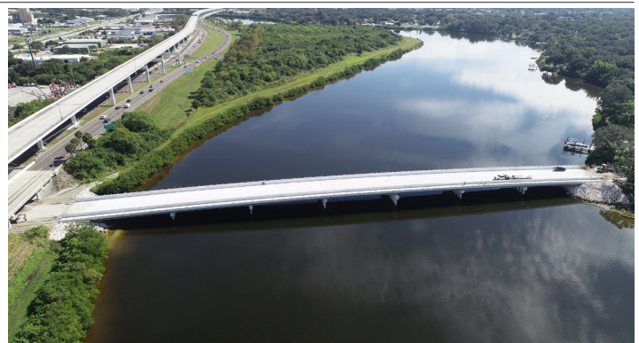
Maydell Drive Bridge: after construction
