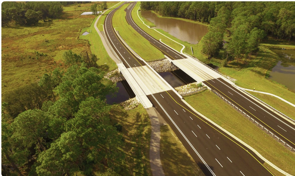
SR 56: after construction
