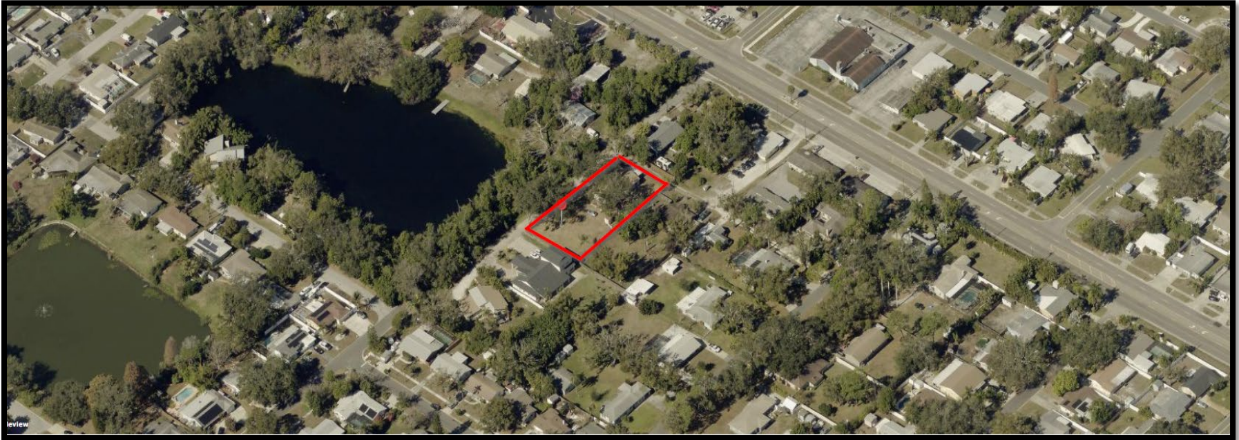
Aerial overview of subject property
