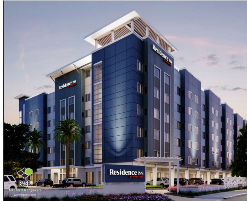
Residence Inn by Marriott Exterior Example
