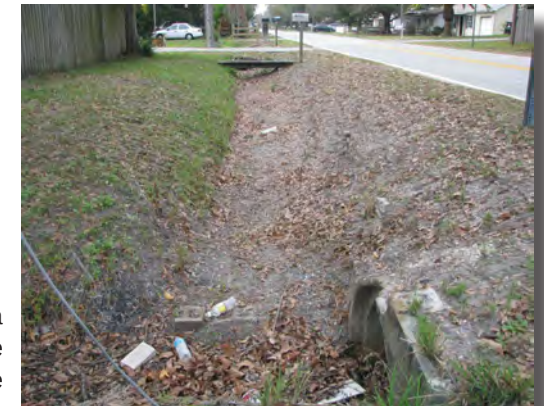
Existing Area Drainage Infrastructure
