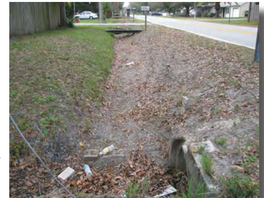
Existing Area Drainage Infrastructure
