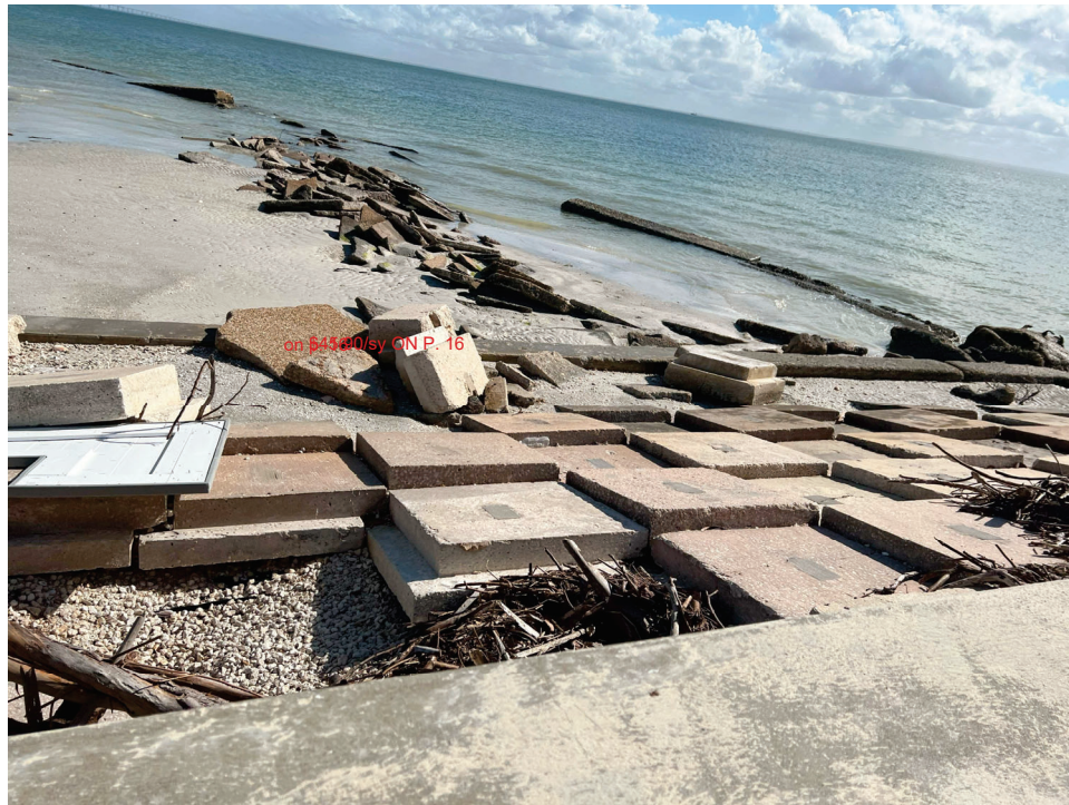
Figure 2-7 Cracked and Displaced Concrete tiles along the seaward side of the Seawall
