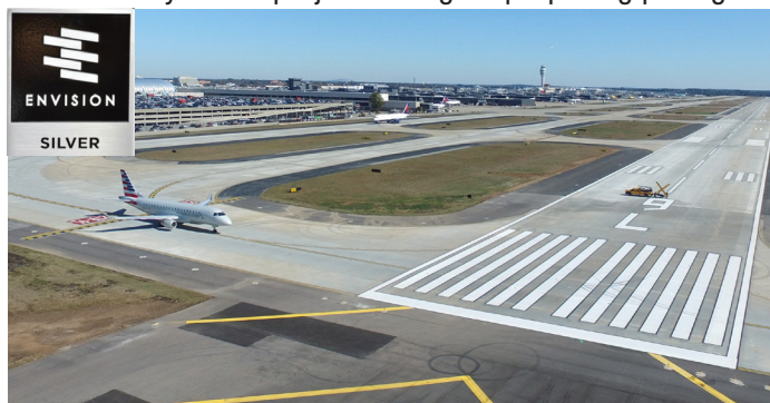
Michael Baker has been involved in multiple projects at ATL (Hartsfield-Jackson International Airport) pursuing Envision certifications, including the most recent Taxiway Pavement Replacement 2019 project that achieved a Silver Award.
