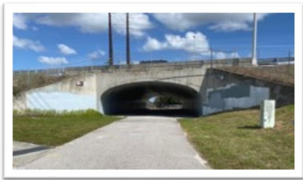
East Entryway, Tarpon Springs
