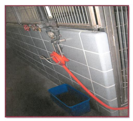
3. Broken tiles. In all kennels, we observed broken tiles under almost all dog pens. The tile supports the bottom of the pens, and in some areas, the tile was very worn, cracked, and chipped. In some of the canine pens, the concrete was deteriorating and exposing the rebar.
