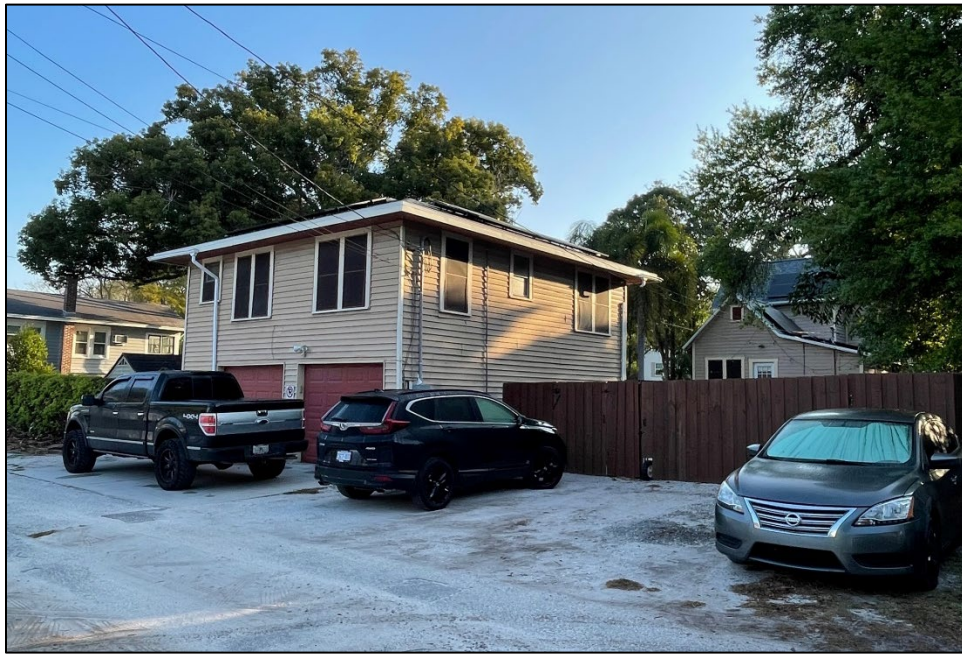
Figure 4: The historic garage apartment building in the rear also had panels installed.
