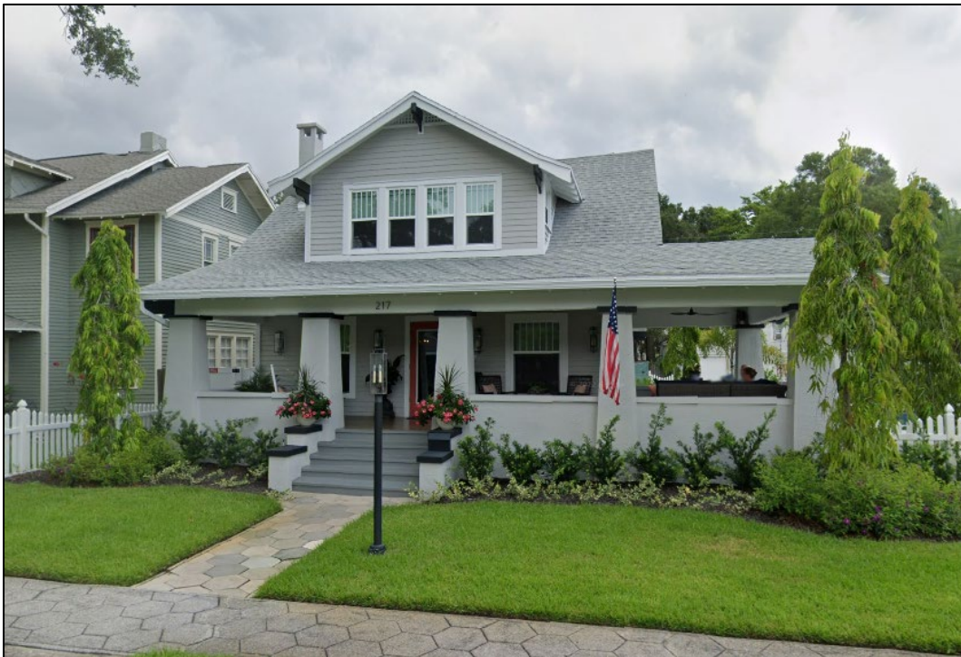
Figure 8: Front elevation after porch rehabilitation. Front porch has been reopened.
