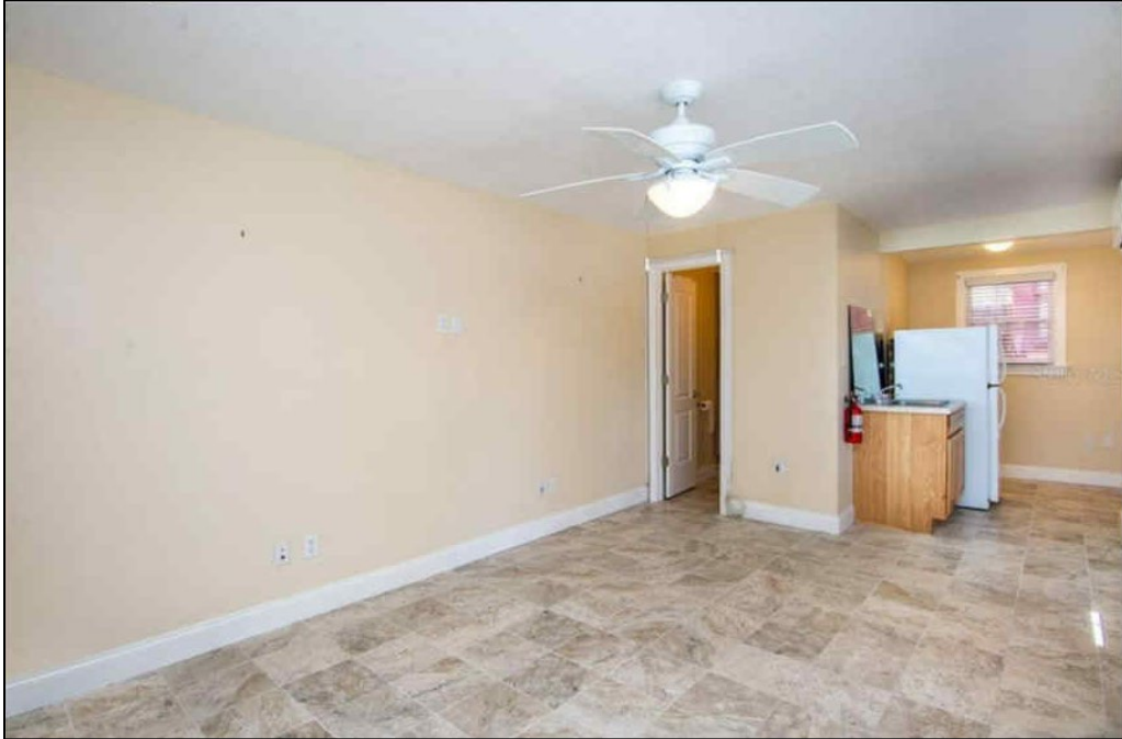
Figure 11: Rear building, studio apartment
