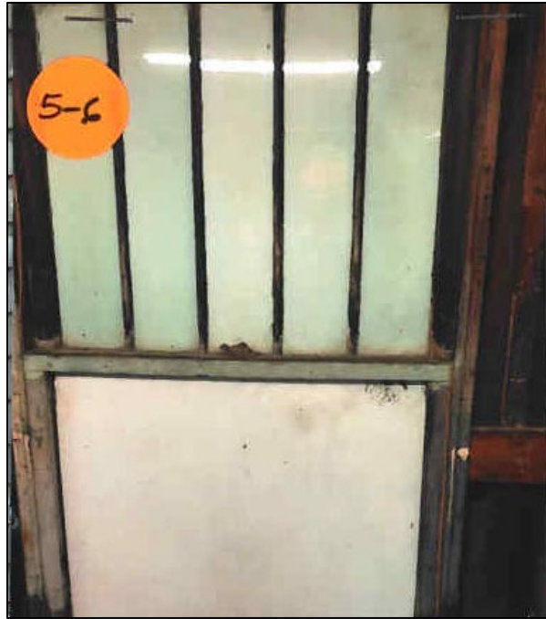
Figure 7: Window to be replaced with new impact window to replicate configuration Appendix B: Post-Construction Photographs (2022)
