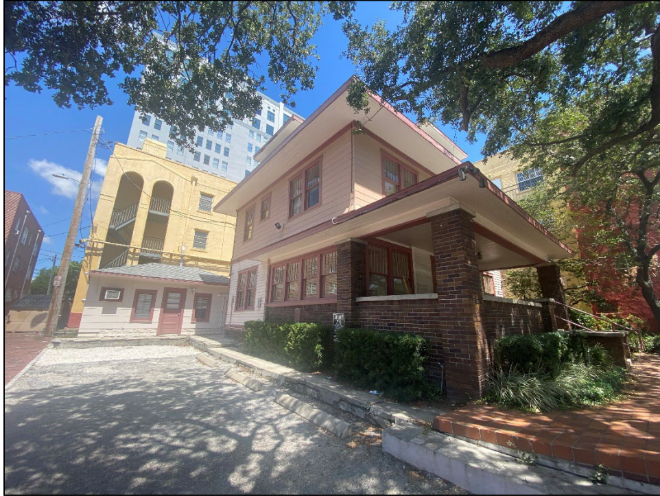
Figure 3: Alley-facing façade and rear structure
