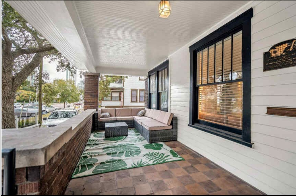
Figure 1: Rehabilitated front porch with original tile
