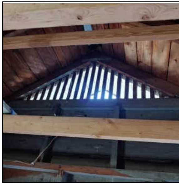
Figure 4: Interior photograph of historic gable vent
