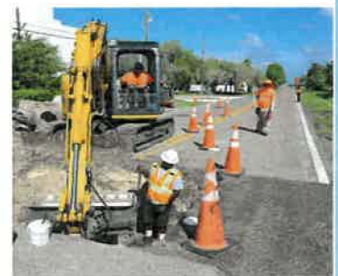
Resurfacing more lanes
