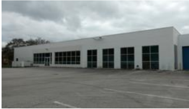
9. Bldg. B – Office space looking SE
