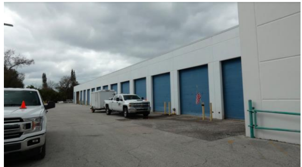
12. Bldg. B industrial space
