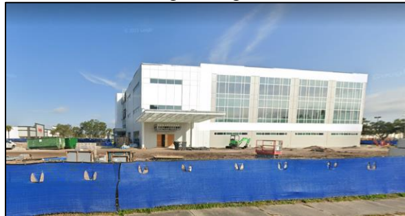
New building during construction
