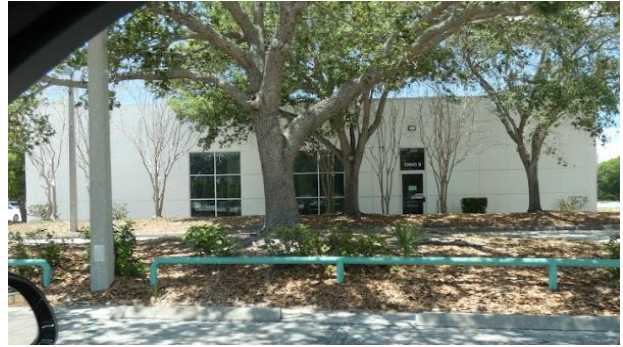
10. Bldg. B office space looking west
