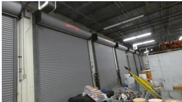
31. Typical Bldg. B overhead doors
