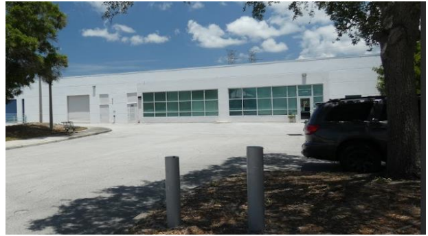
8. Bldg. B – Office space
