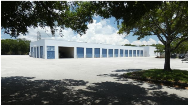
7. Bldg. B – Industrial space
