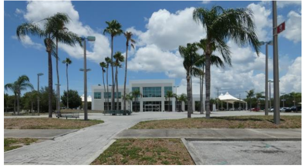
2. View north toward Building
