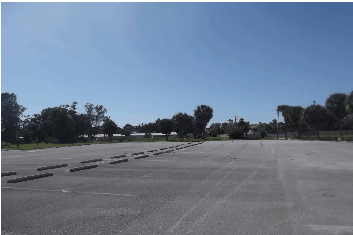
PARKING AREA VIEW SOUTH
