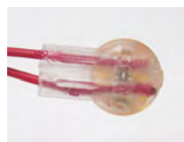
Figure 63: Wires in gel cap
