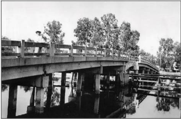
Figure 1. Beckett Bridge in 1965, facing Southwest
