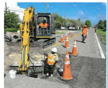
Resurfacing more lanes
